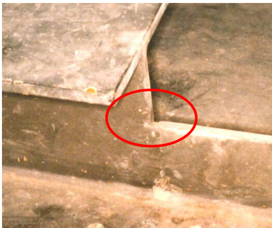
Figure 85. Photo. Bad coped beam detail with a sharp corner (left) and better coped detail with a smooth ground transition radius (right).
