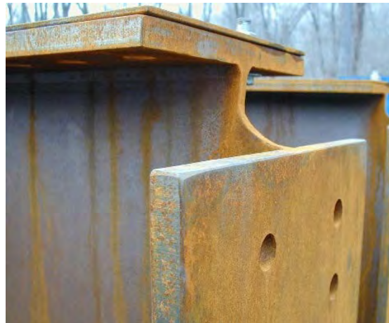
Figure 85. Photo. Bad coped beam detail with a sharp corner (left) and better coped detail with a smooth ground transition radius (right).
