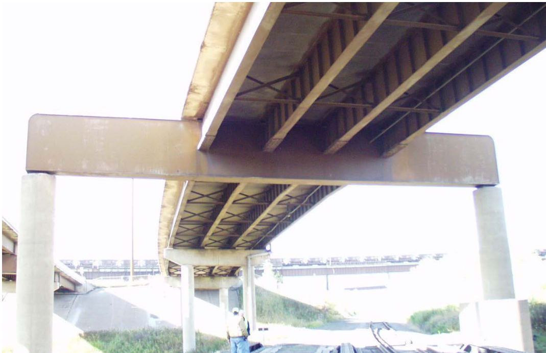
Figure 89. Photo. Picture of MnDOT bridge #69832 in Duluth, Minnesota.
