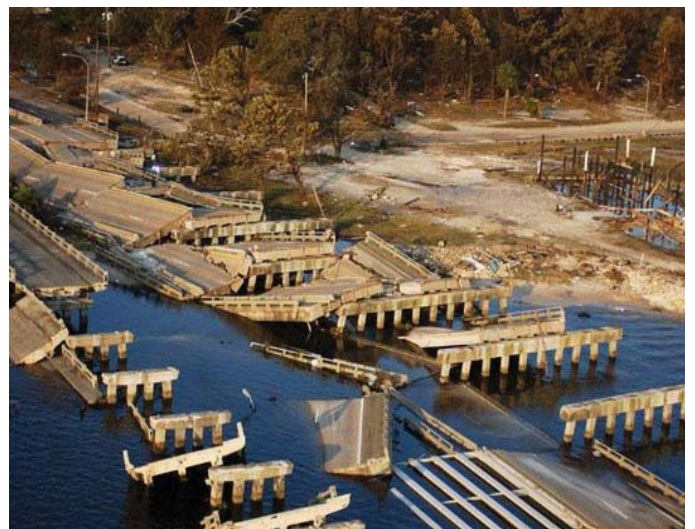
U.S. 90 Ocean Springs bridge. (2005)
