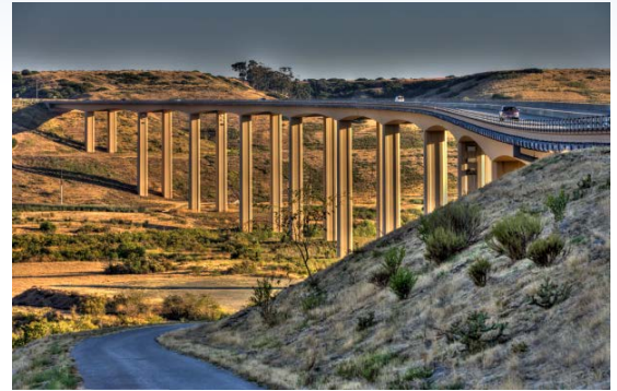
Bridge on the South Bay Expressway, a 10-mile toll road that helps link San Diego's highway network with Otay Mesa, the region's main commercial Port of Entry
