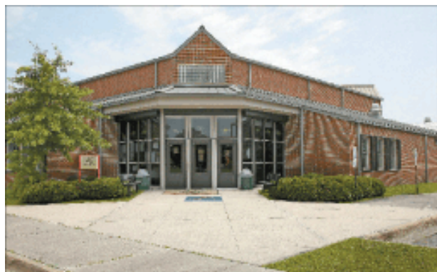
Cherry Tree House: Bldg. 4415 "C" Street (252) 466-3769
