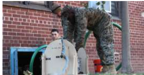
Marines with 8th ESB, 2nd MLG get ready to start a gas-powered pump to remove water from a flooded basement while conducting humanitarian operations in Far Rockaway, N.Y., Nov. 4. Approximately 86 Marines from the unit were deployed to New York to help pump water from flooded areas of the state. (Photo by LCpl Scott W. Whiting)
