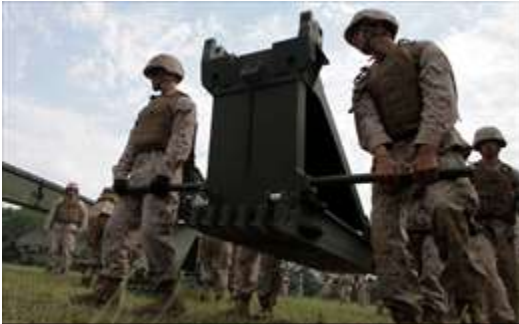
Photo Marines with 6th ESB use a team-lift technique to move a 300 pound piece of bridge equipment during a training exercise here, June 11. Many of the pieces used to put together a medium girder bridge require more than one Marine to effectively move them. (Photo by Cpl John M. McCall)
