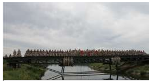
Marines with Bridge Companies A, B and C, 6th ESB pose atop a medium girder bridge during a training exercise here, June 11. These Marines worked together late into the night in order to complete the project in a single day. (Photo by Cpl John M. McCall)
