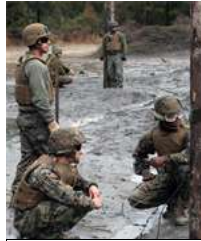
Marines with the units set explosives in a tree, a part of a timber charge that can be used to clear trees to make a path. Photo by: Lance Cpl. Phillip R. Clark
