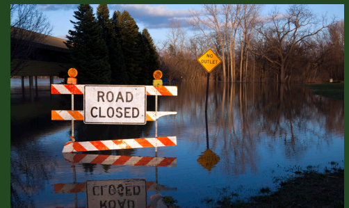
Flooded parking lot in Michigan. Photo credit: MDOT
