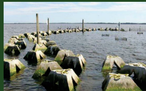
Wave Attenuating Devices. Photo credit: Scott L. Douglass, University of South Alabama (credited to Lamb, 2006)
