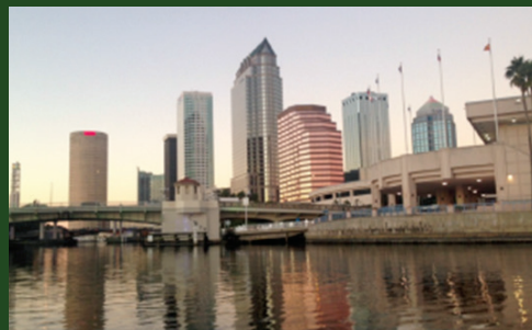
Downtown Tampa. Photo credit: Jacobs Engineering, 2014
