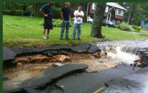
Severe roadway damage during a storm. Photo credit: Foothills Media Group, 2011.
