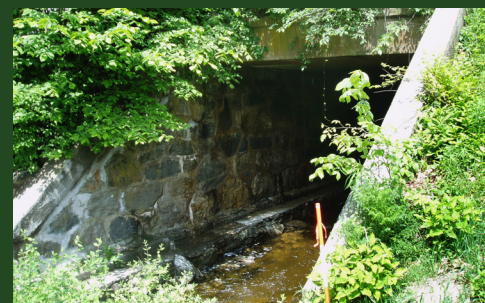
Culvert with surrounding vegetation. Photo credit: ConnDot Hydraulics and Drainage Section.
