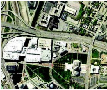
An aerial image of the I-95 Northbound Viaduct Replacement site in Providence, RI.
