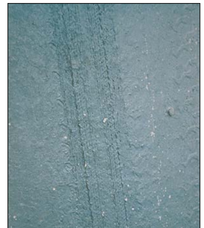
FIGURE 38 Distress Type ACP 11—Aggregate Obscured.
