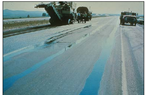
FIGURE 33 Distress Type ACP 9—Standing Water in Ruts.
