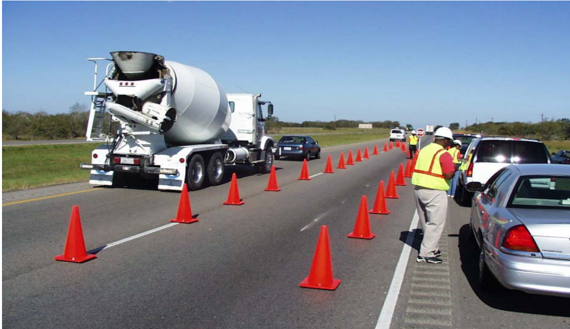
Figure 12: External Station Survey
