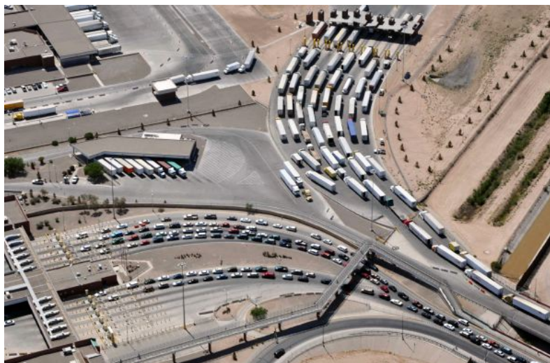
Figure 25: Zaragosa Bridge (El Paso, Texas)
