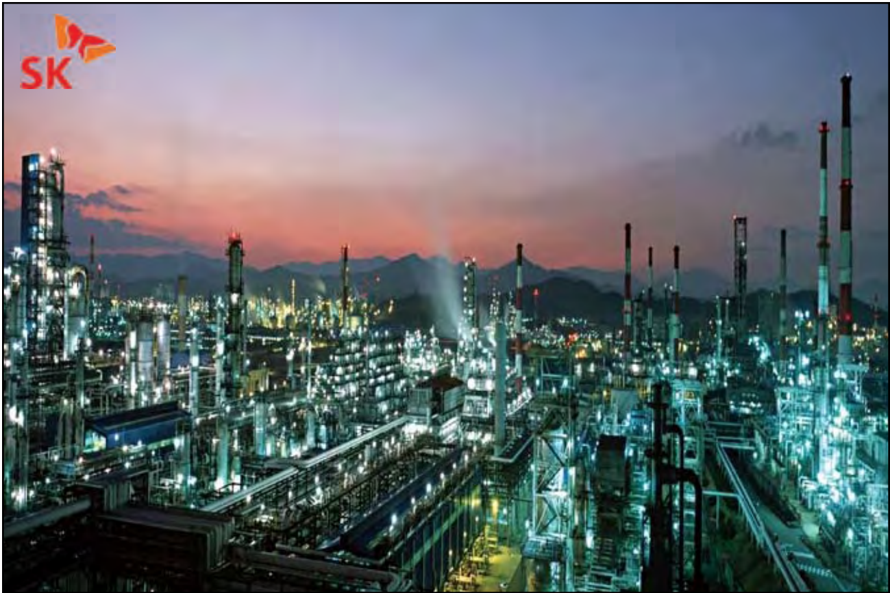
SK oil refinery in Ulsan, southeast Korea. SK Energy is Korea's largest energy company, and its Ulsan refinery is one of the largest such facilities in the world. (Photo by SK)
