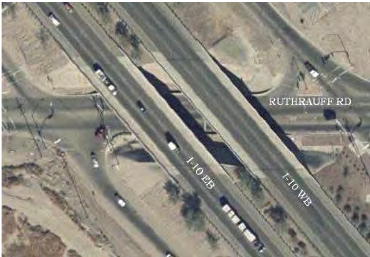
Figure 1-1. Aerial view of a pair of 3-span Interstate 10 (I-10) bridges over a local roadway in Tucson, Arizona.
