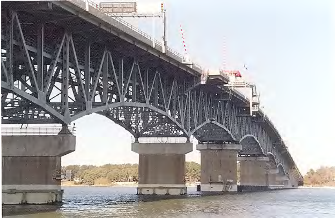
Figure 1-4. A major multi-span bridge structure over water (George P. Coleman Bridge over the York River in Yorktown, Virginia).
