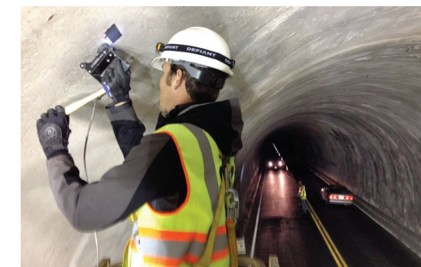
Nondestructive Testing for Tunnel Linings (R06G) | Photo courtesy Olson Engineering
