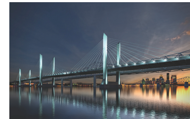
Service Life Design for Bridges (R19A) | Photo courtesy KYTC
