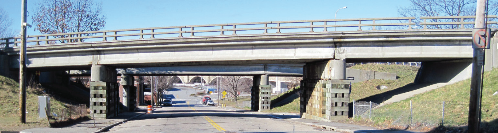
Rhode Island DOT replaced and reopened the Warren Avenue Bridge in just 21 days using Innovative Bridge Designs for Rapid Renewal . | Photo courtesy RIDOT
