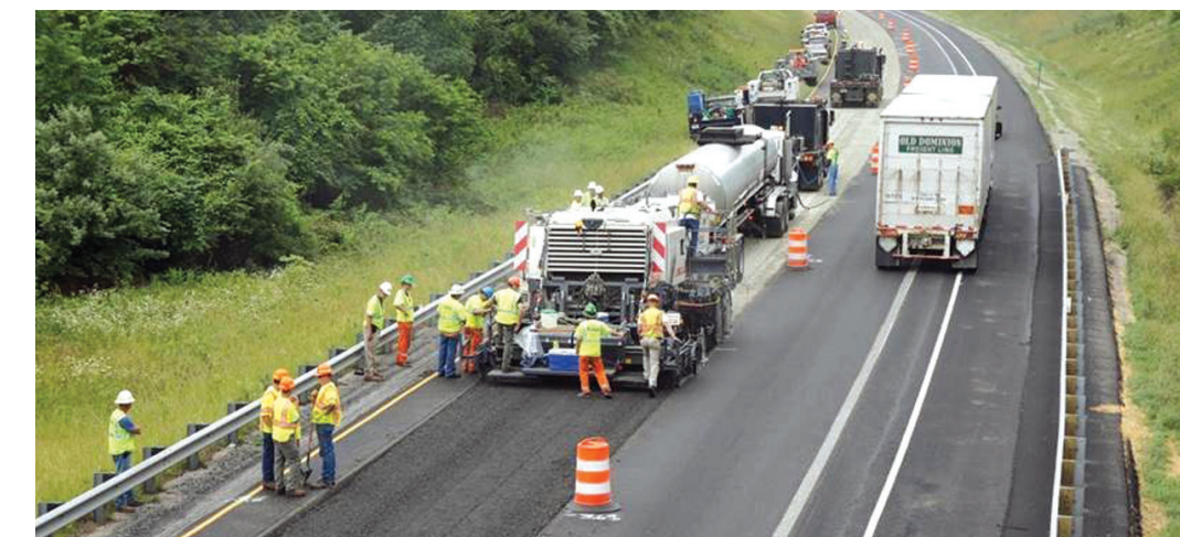
A pavement recycling operation in Virginia. | Photo courtesy VDOT
