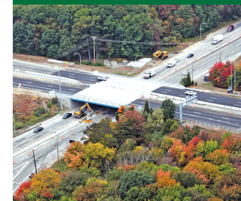
The completed Warren Ave Bridge, Providence, RI | Photo courtesy RIDOT
