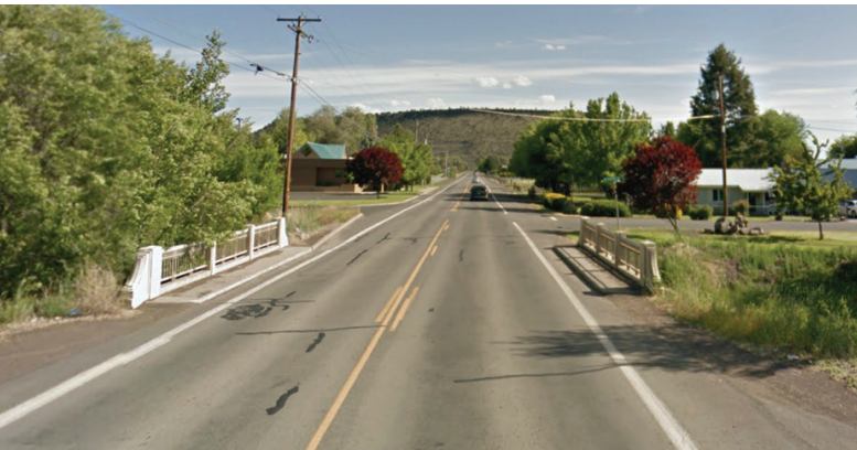
The Ochocho Creek Bridge in Prineville, OR that will be replaced using Managing Risk in Rapid Renewal Projects . | Photo courtesy Lea Ann Hart-Chambers, Oregon DOT
