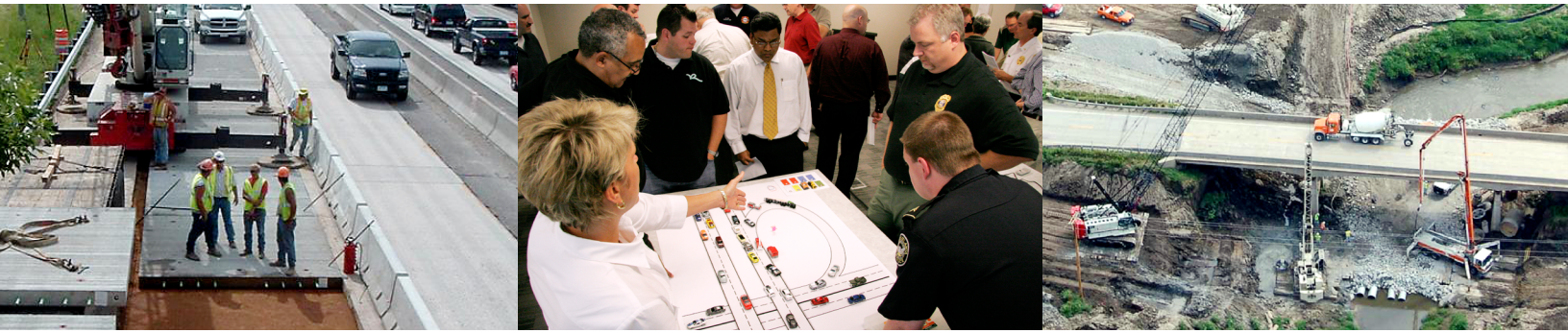
Photos from left to right: Workers position a slab of precast concrete pavement; First responders study traffic incident scenarios as part of a training pilot held in Georgia; An accelerated bridge construction project over Keg Creek in Iowa.
