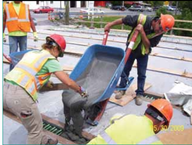
Figure 1. Placement of UHPC into longitudinal connection between deck-bulb-tee girders.
