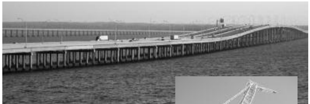
The new I-10 Escambia Bay Bridge in Pensacola, FL. The bridge was reconstructed in 63 days after being destroyed by Hurricane Ivan in 2004.
