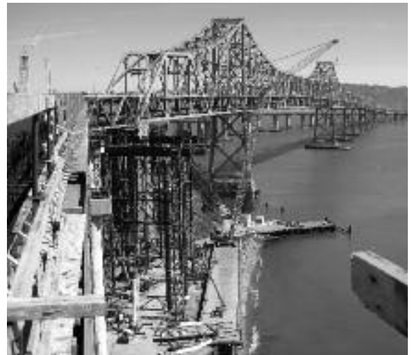
Accelerated construction practices being used as part of California's San Francisco-Oakland East Bay Bridge project include a planned replacement of a 91-m-long (300 ft) double-deck section of the bridge's East span over Labor Day weekend in September 2009.
