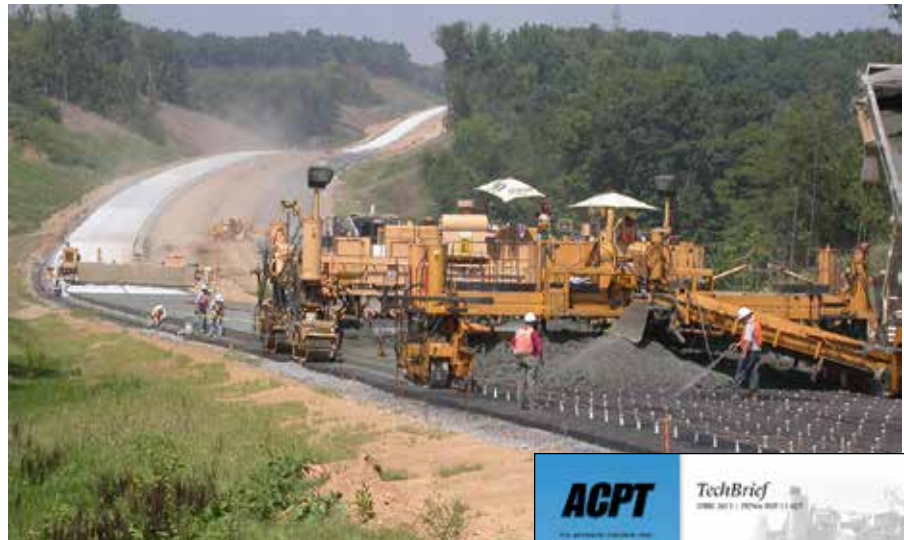
Continuously reinforced concrete pavement can extend joint free for many miles and has low maintenance requirements.
