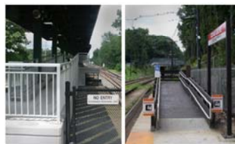
Mini-High Platform with Appropriate Barrier
