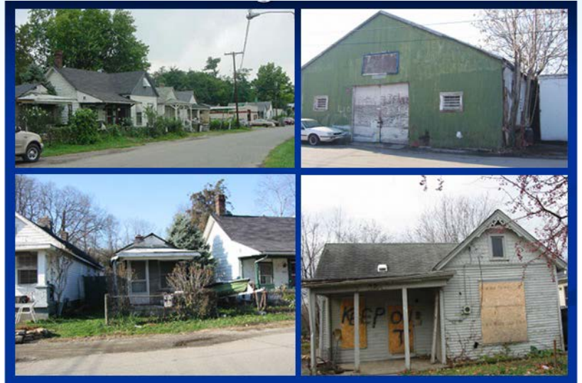
Figure 2: Davis Bottoms before implementation of the redevelopment plan
