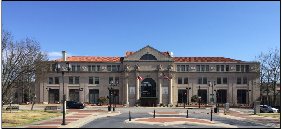
Figure 4: Macon’s historic 100-year-old Terminal Station, home to the Macon-Bibb County Transit Authority, the city’s central bus terminal. It may soon serve passenger rail (Image courtesy of Chris Floore, Macon-Bibb County).
