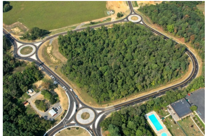
Figure 3: NJDOT constructed an innovative design featuring a series of roundabouts that slow traffic and better distribute flow. (Image courtesy of contextsensitivesolutions.org)
