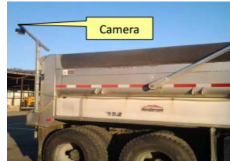
Figure 14: Rear view camera system installations won an Operations Best Practices Award. (Image courtesy of NYSDOT)
