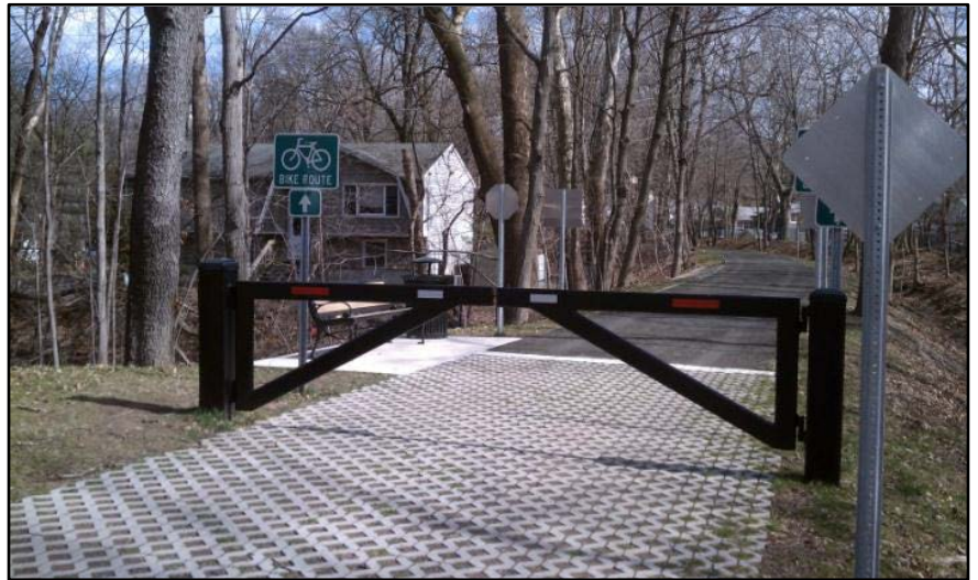
Figure 4: Permeable pavements allow stormwater to infiltrate, mitigating the hydrologic impacts of transportation infrastructure.
