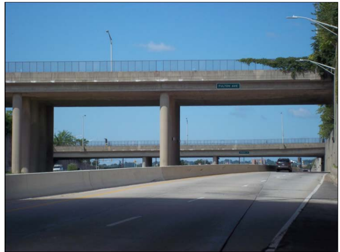
Figure 1: Fulton Avenue Bridge spans the "highway to nowhere" and connects bisected West Baltimore neighborhood (Image courtesy of FHWA).
