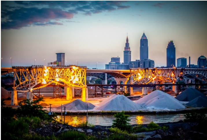
Figure 3: The steel skeleton of the old Innerbelt Bridge was demolished using explosives in July 2014. In total, 19,775 tons of steel and steel rebar were recycled from the old bridge. (Image courtesy of Marianne Mangan)
