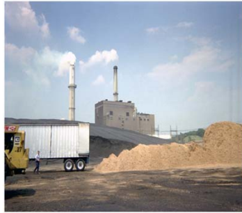
NIPSCO generating station
