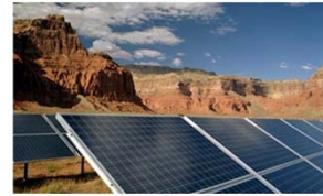
Photo by Warren Gretz, NREL 08024
