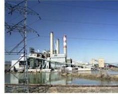
Electrical transmission lines in front of coal-fired power plant Photographer: Warren Getz Source: NREL photo library 10933.jpg
