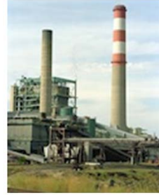
Cherokee Station coal-powered plant, Denver, Colorado Photographer: Warren Getz Source: NREL photo library 06360.jpg
