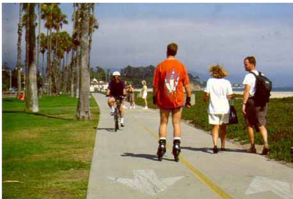
Figure 19-1. Photo. To minimize user conflicts, adequate trail width is critical on paths having high volumes and diverse user mixes (Santa Barbara, CA).
