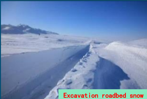
Half filling and half digging of snow
