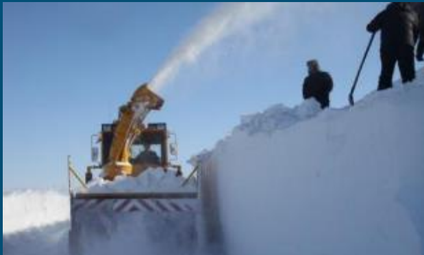
Half filling and half digging of snow
