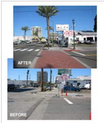
Streetscaping in Oakland | Metropolitan Transportation Commission Transportation for Livable Communities Program
