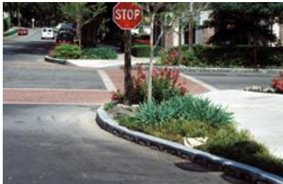
Intersection with bulb-out | Claremont CA
