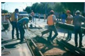
NJ FIT Light Rail Construction | New Jersey DOT
