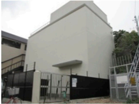
Ventilation Outlet located between Kitasenju and Machiya on Chiyoda Line
