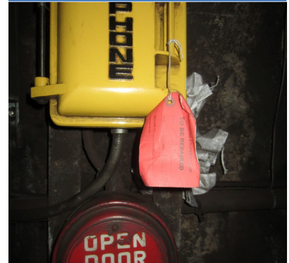
Broken communication gear
