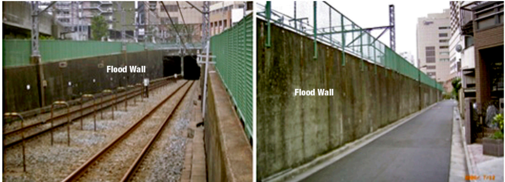
Flood Wall at the Kitasenju Outlet of the Chiyoda Line Tunnel
