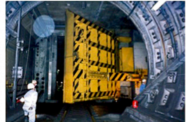
Flood Gate in a Tube
