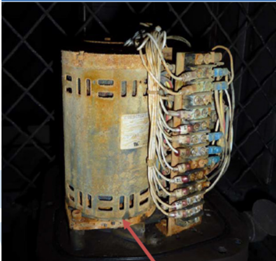
Damaged fan control
