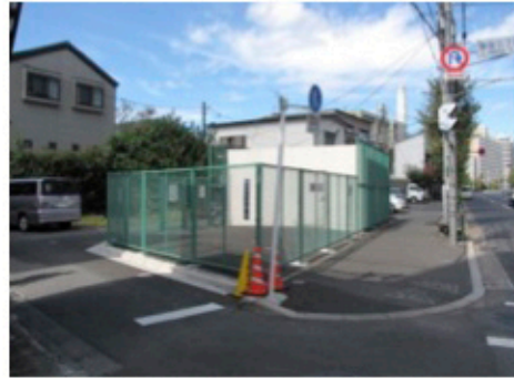
Ventilation Outlet located between Ojikamiya and Shimo on Nanboku Line
