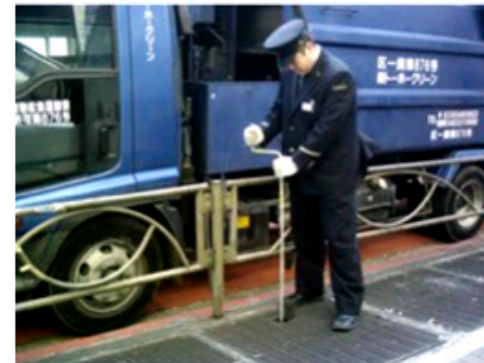
Manual Operation in Case of Malfunction of Automatic Shutter
