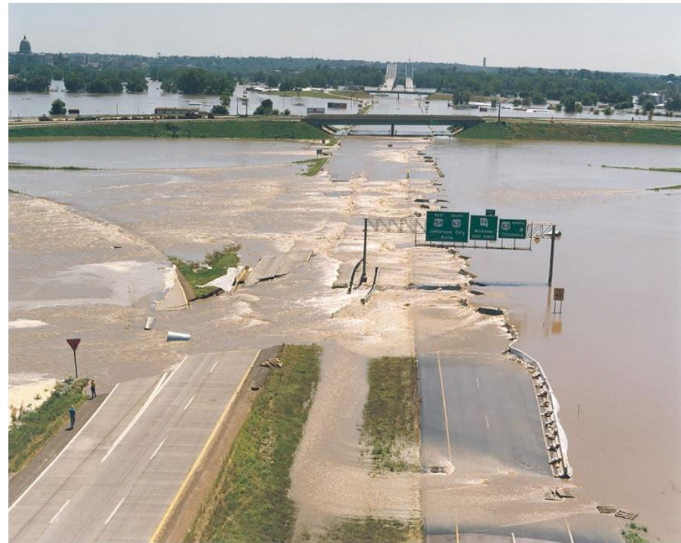
Missouri River flooding, Jefferson City, Missouri Photo: Missouri DOT
