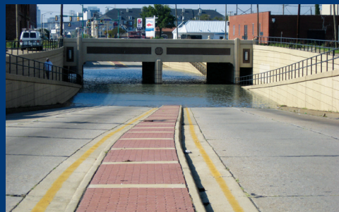
Flooding of the Monticello Avenue underpass in Norfolk, VA. Photo credit: City of Norfolk
