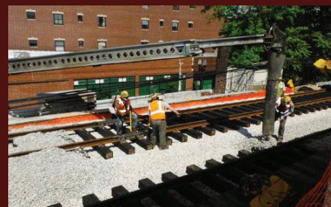
Ballasted track structure construction. Photo credit: CTA.
