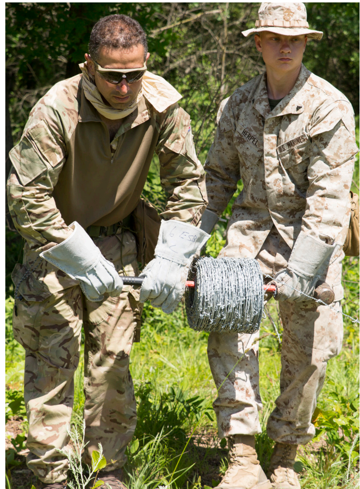
Lance Cpl. Robert L Herpel (right), a combat engineer with Company C, 6th Engineer Support Battalion, 4th Marine Logistics Group, and Pvt. Antonio Comparetto (left), a sapper with 131 Commando Squadron Royal Engineers, British army, unwind barbed wire to build a defensive obstacle during exercise Red Dagger at Fort Indiantown Gap, Penn., June 13.
