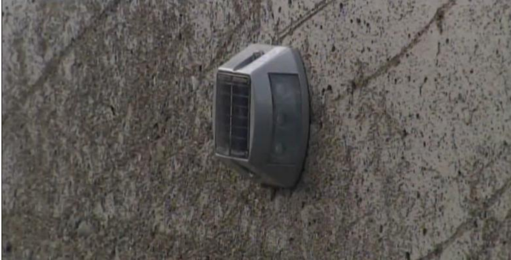
Figure 15. Photo. LED barrier delineator used for the I-90 project.
