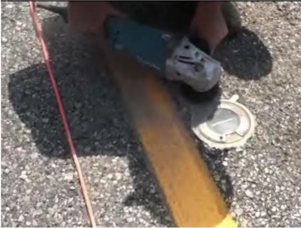
Figure 7. Photo. Grinding relief in front of the base of lane marker.
