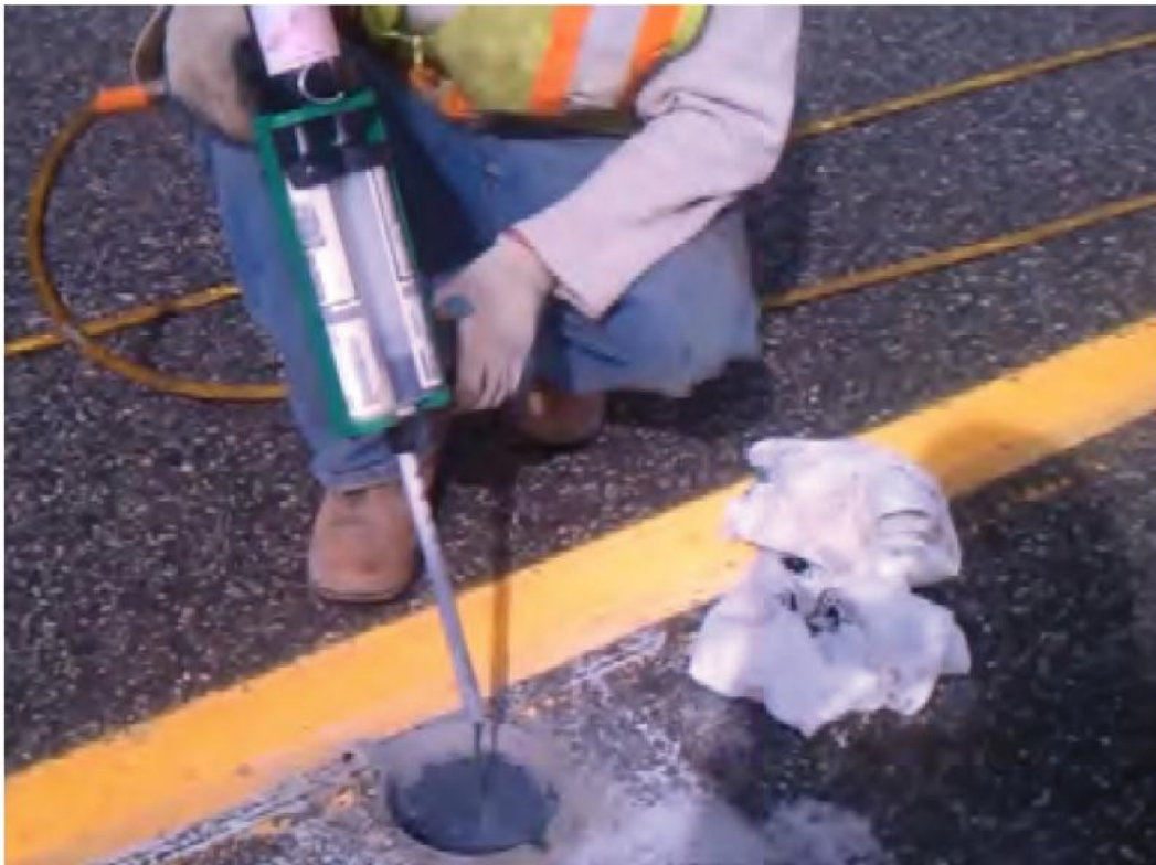
Figure 4. Photo. Filling the bottom of the hole with epoxy.
