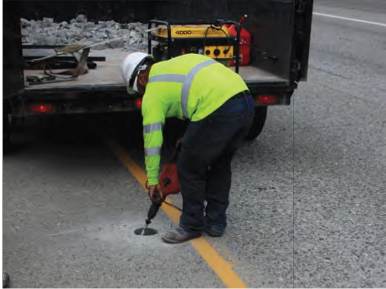
Figure 3. Photo. Drilling a hole into the pavement for the LED delineator.
