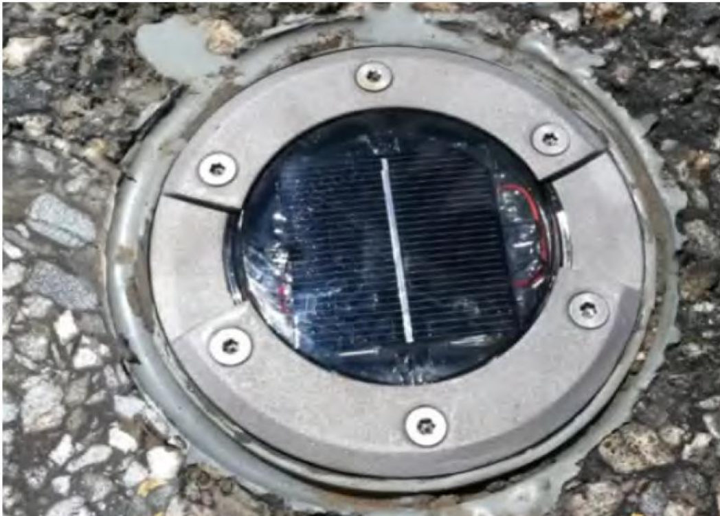
Figure 8. Photo. Inserting and securing the LED into the base.
