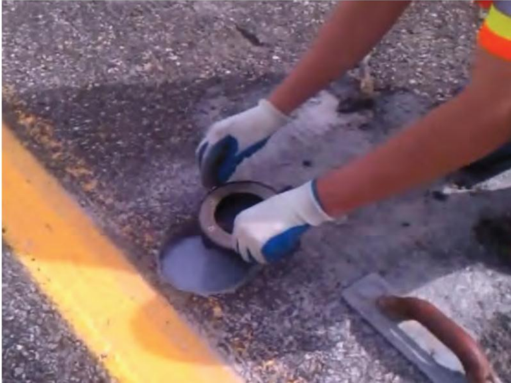
Figure 5. Photo. Aligning the base of marker into the hole.
