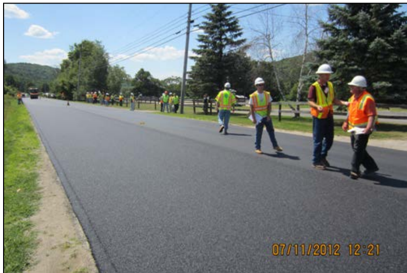
Figure 42. Participants and construction team members inspecting the longitudinal construction joint.
