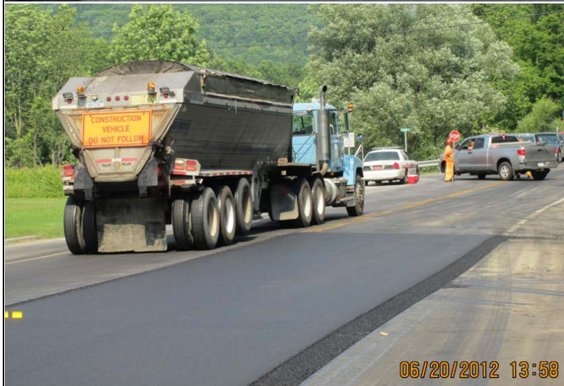
Figure 10. Trucks used to deliver the HMA and WMA mixtures to the paver.
