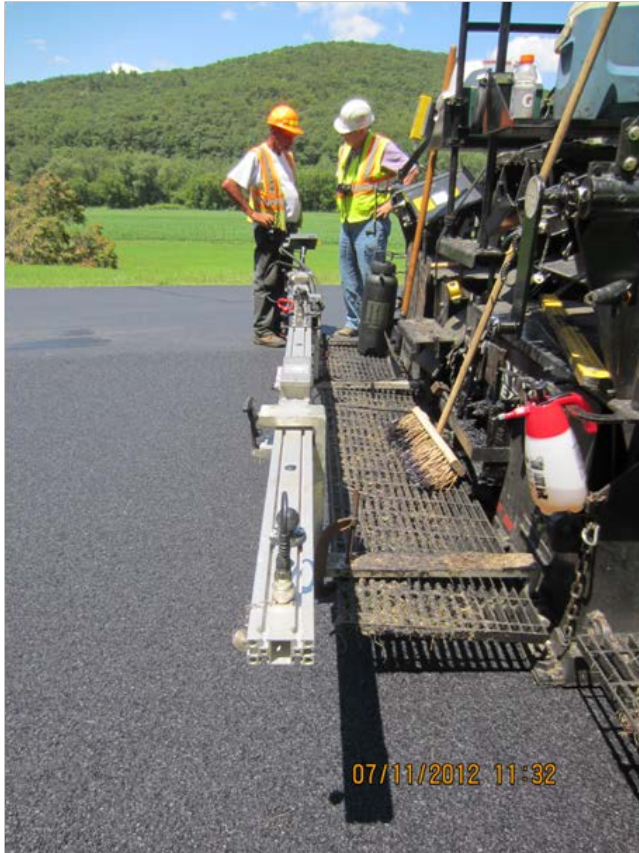
Figure 41. Participants viewing the mat surface temperatures displayed on the screen of the IR bar attached to the platform behind the screed.
