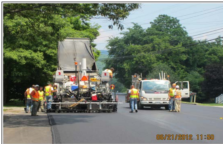
Figure 12. Overhanging trees and power lines along U.S. 4A in Castleton.
