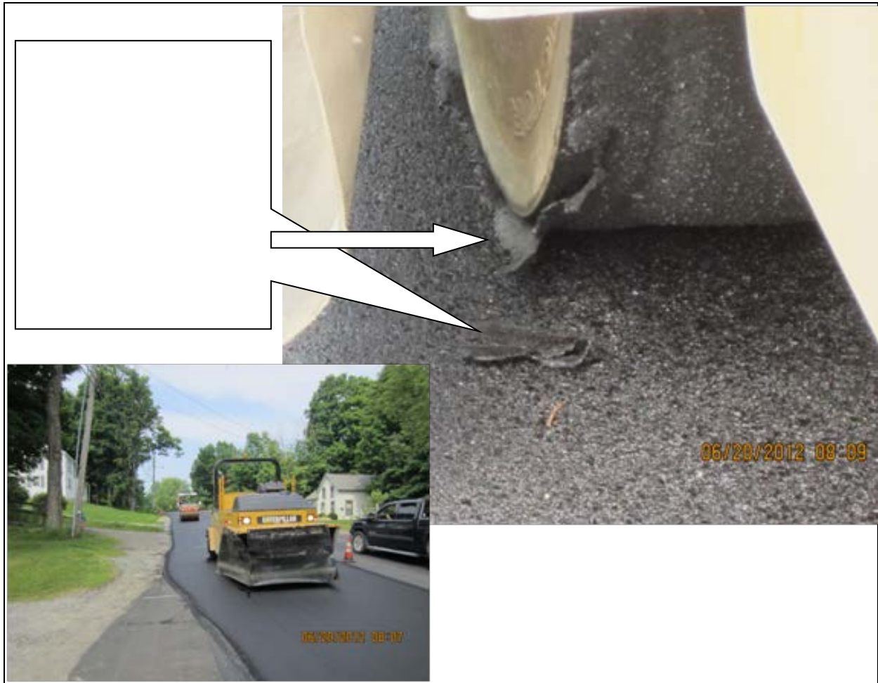
Figure 32. Rubber tires picking up the mastic from the WMA surface.
