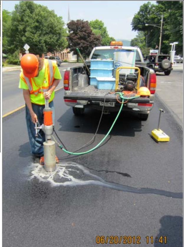
16b. Drilling cores in the WMA mat for acceptance.
