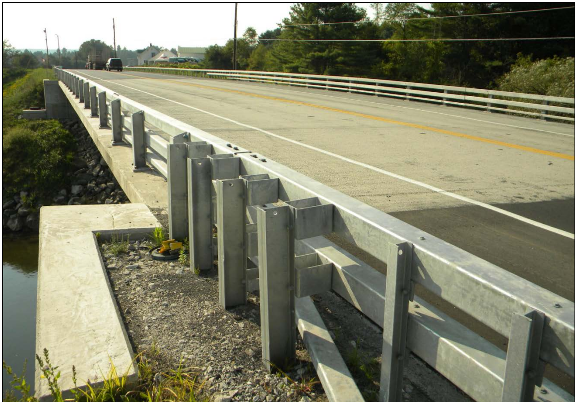
Figure 29. Roadside view of the completed bridge.
