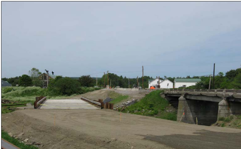
Figure 17. Construction of two-way temporary bypass bridge.
