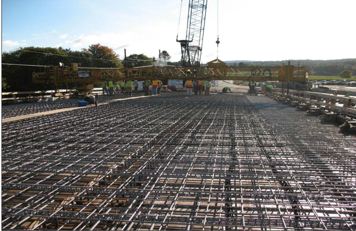
Figure 24. View of deck reinforcement.
