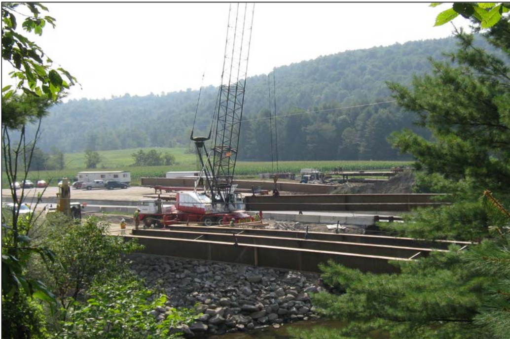
Figure 19. Placement of weathering steel girders.
