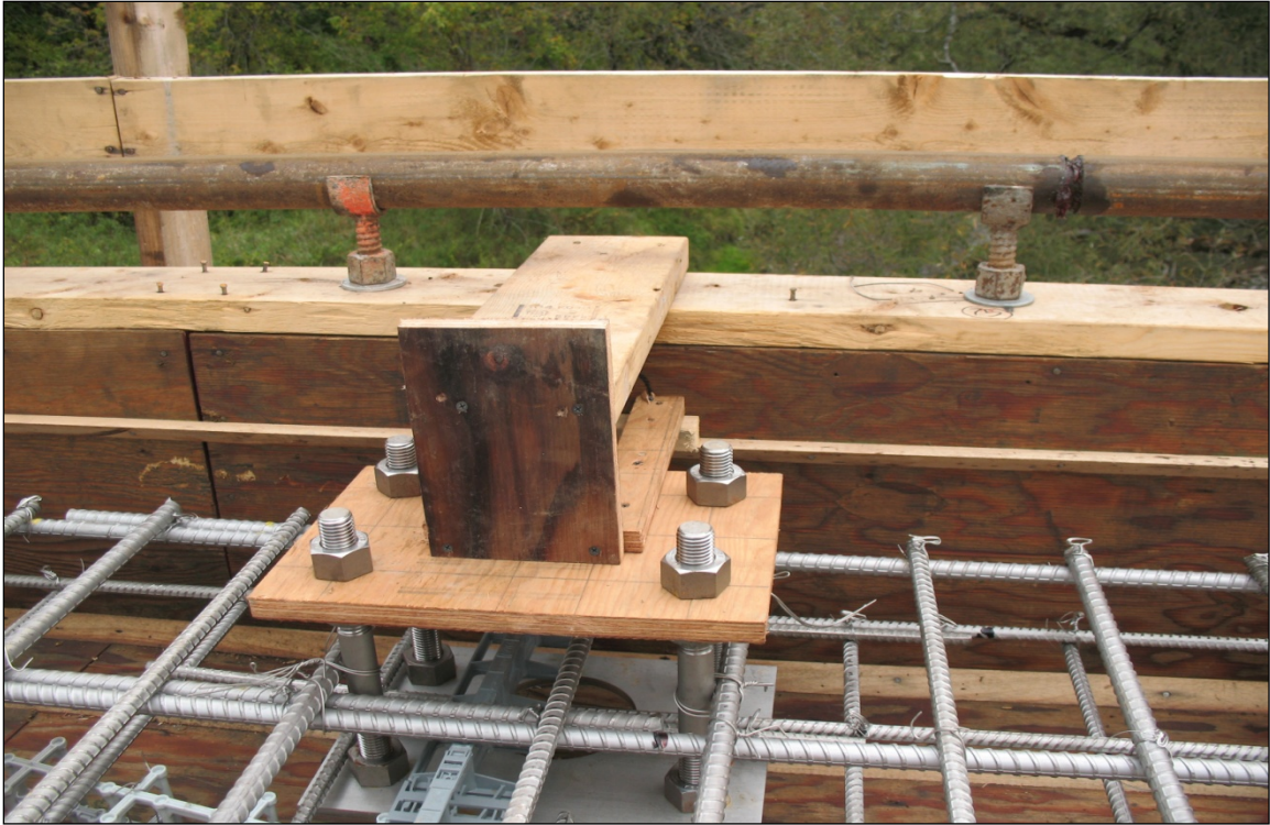
Figure 26. Anchor bolt assembly detail.
