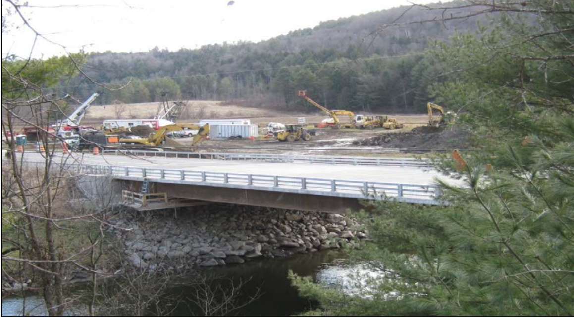
Figure 28. View of the completed bridge.
