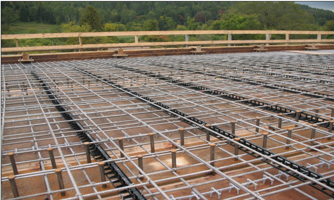
Figure 25. Close-up of deck reinforcement.
