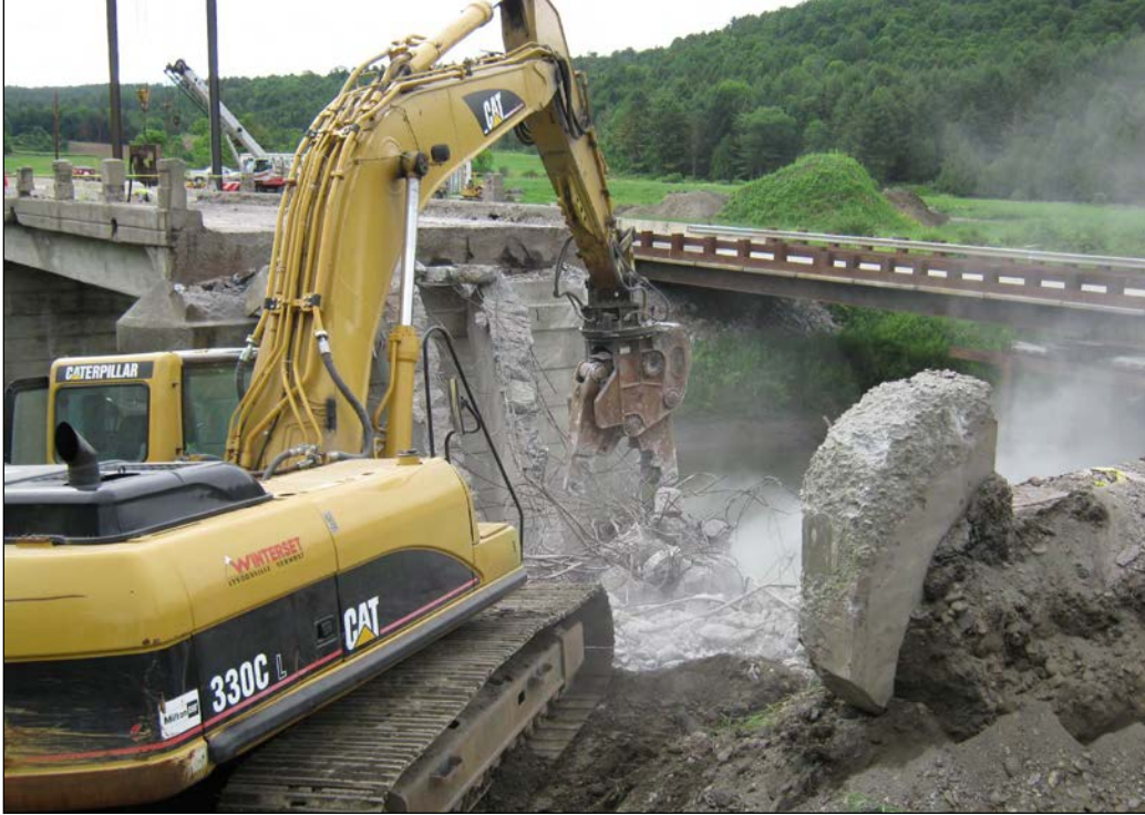
Figure 18. Demolition of the existing bridge.
