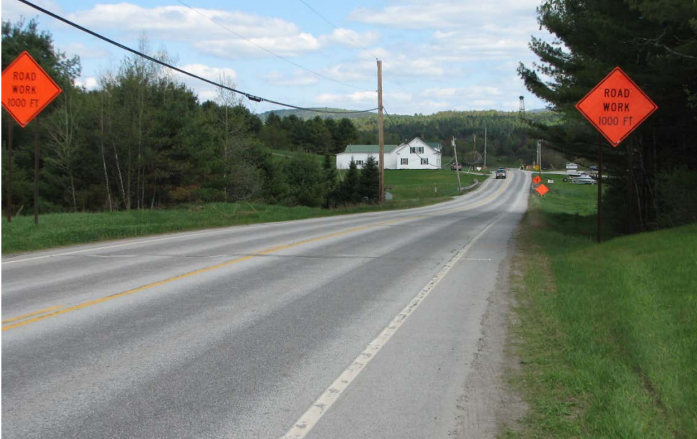
Figure 30. First work zone warning.
