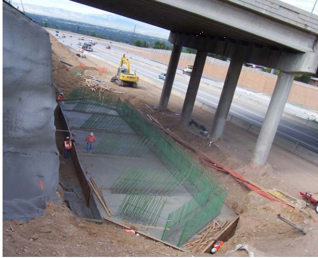
Figure 7. View of the east spread footing.
