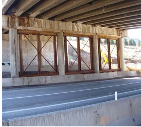
Figure 3. Shoring the bent caps.
