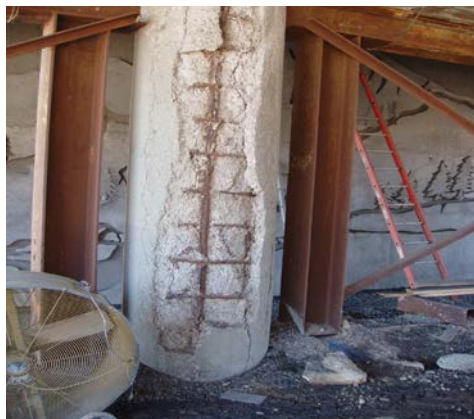
Figure 2. Delaminated column.
