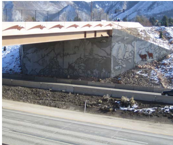
Figure 26. View of the new 4500 South Bridge.
