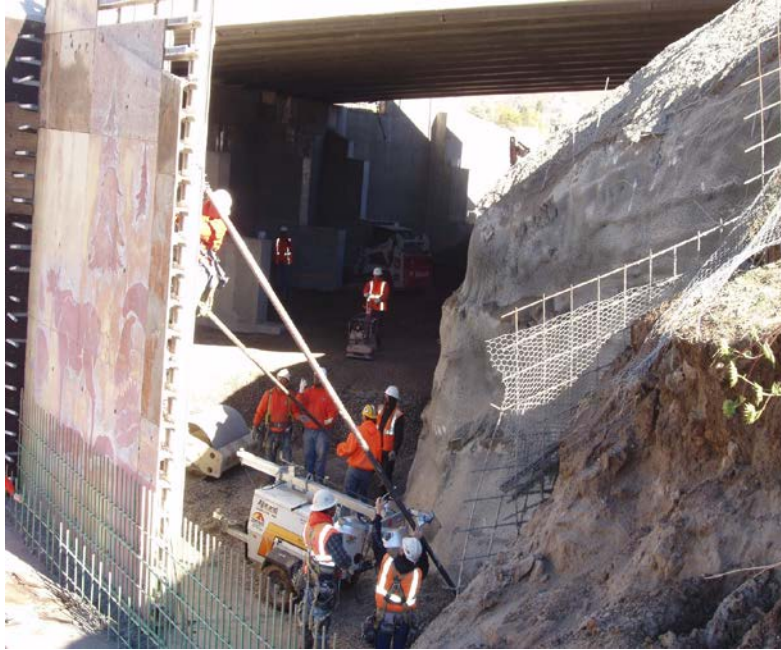
Figure 13. Seating the backfill material.
