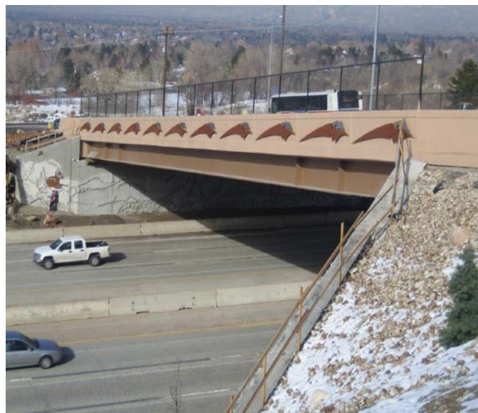
Figure 27. Another view of the new 4500 South Bridge.
