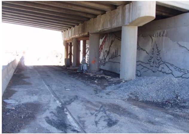
Figure 8. View of the CIP abutment.
