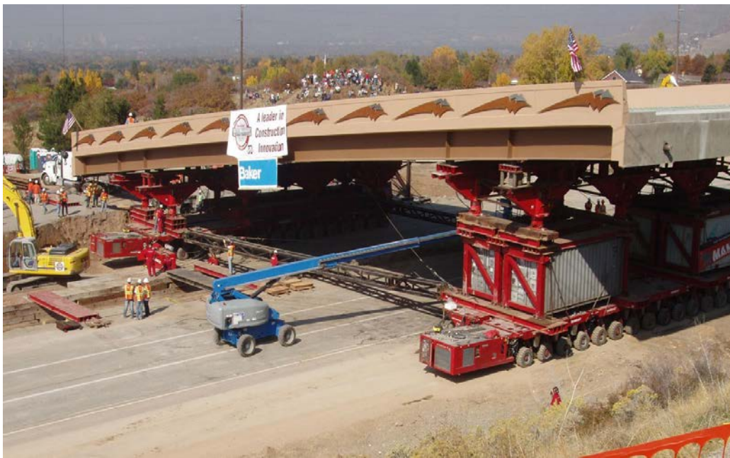
Figure 23. Another view of moving the superstructure.
