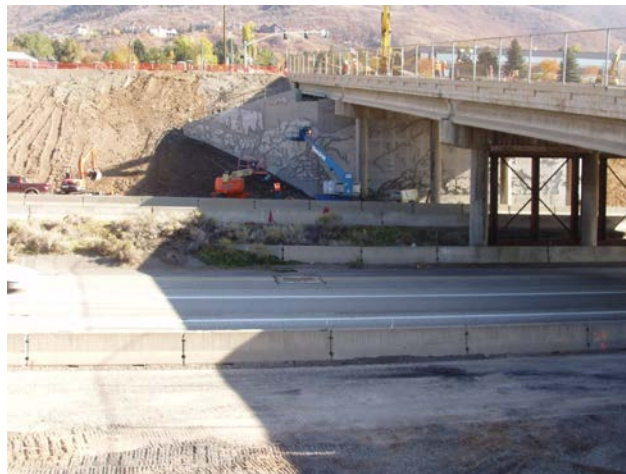
Figure 9. View of CIP wingwall.
