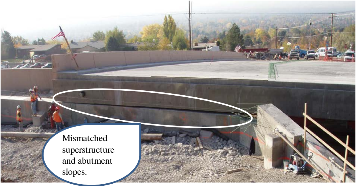
Figure 24. Top view of the deck over the abutments.
