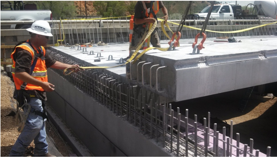
Figure 38. Photo. Bridge deck elements being placed (courtesy: UDOT).
