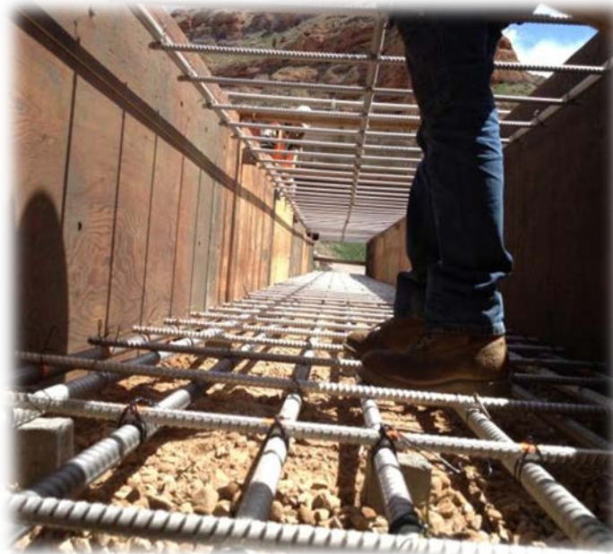
Figure 34. Photo. Bearing sill/footing (courtesy: UDOT).
