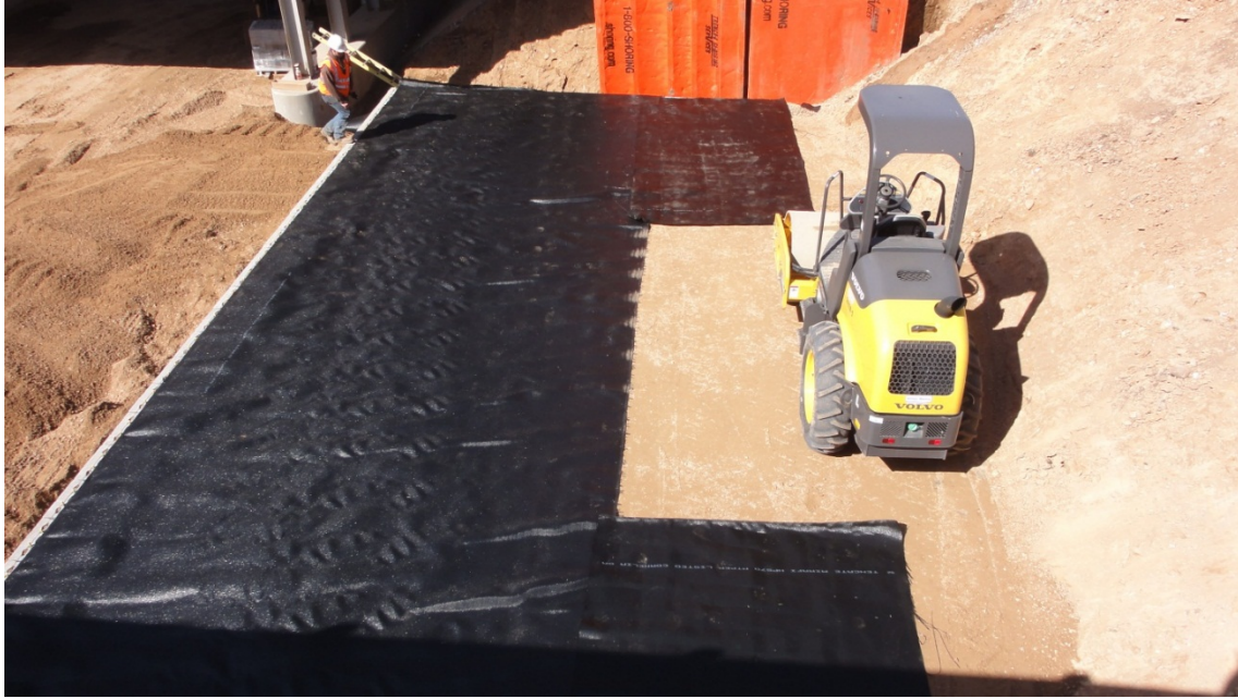
Figure 31. Photo. Geotextile reinforcement placed on the compacted surface.
