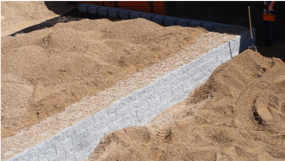
Figure 32. Photo. Granular fill placed on top of the geosynthetic material.
