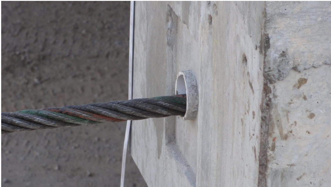
Figure 45. Photo. Cable used for bridge slide.
