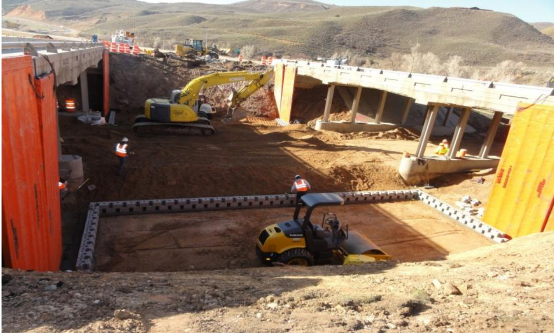
Figure 28. Photo. Two completed courses of SMU blocks.
