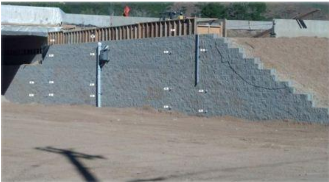
Figure 17. Photo. Survey targets and inclinometers placed on the eastbound bridge wall (courtesy: UDOT)
