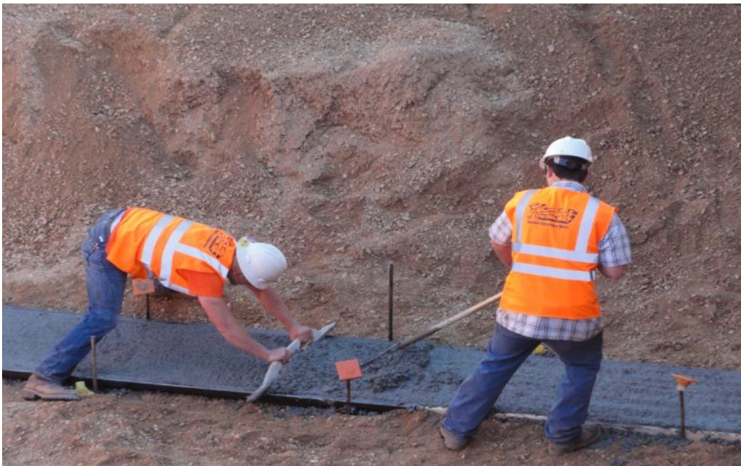
Figure 26. Photo. Preparation of leveling pad.
