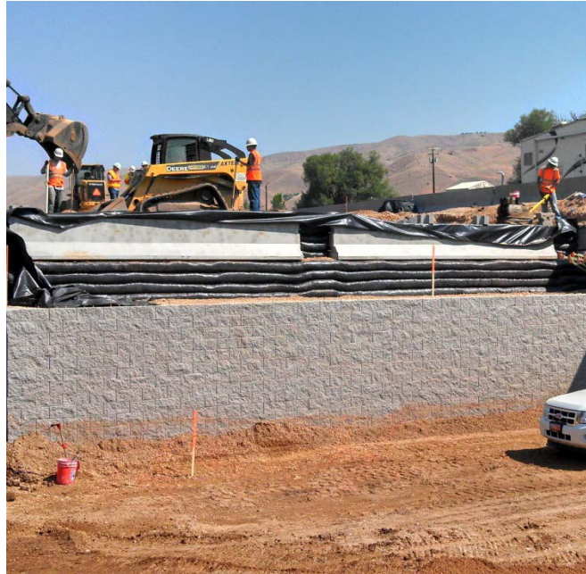
Figure 33. Photo. Top four courses of geotextile-wrapped layers (courtesy: UDOT).
