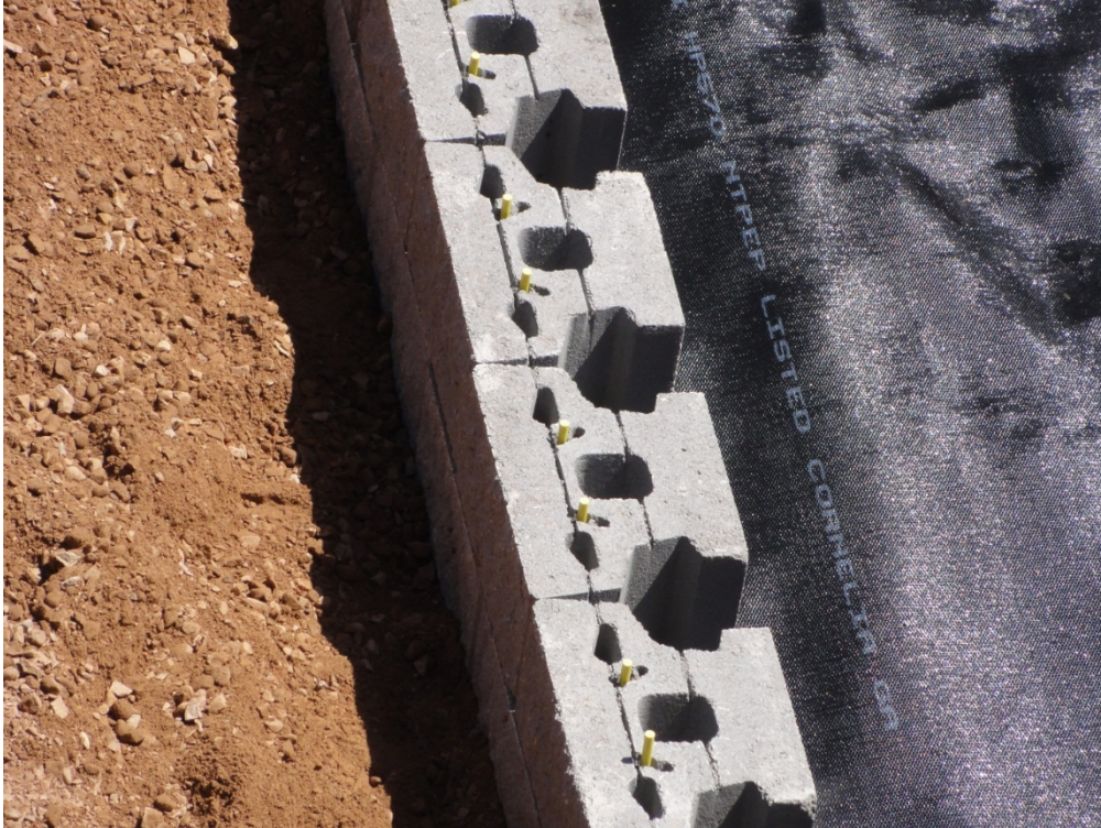
Figure 12. Photo. Segmental block units with fiberglass pins.
