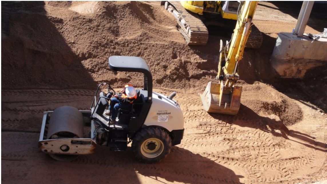
Figure 24. Photo. Roller operations.
