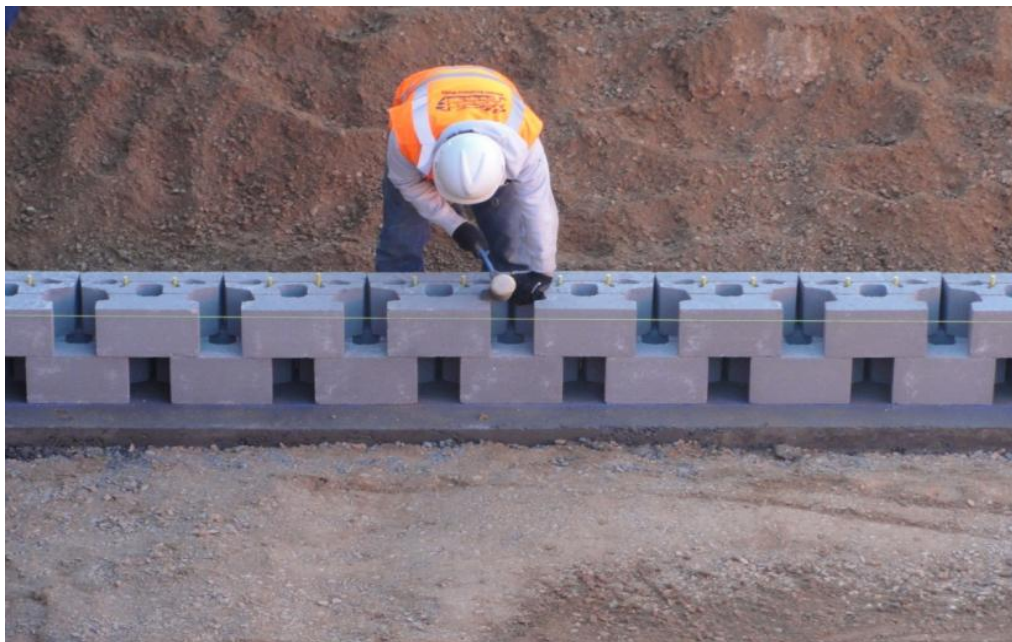
Figure 27. Photo. Aligning the second course of SMU blocks.
