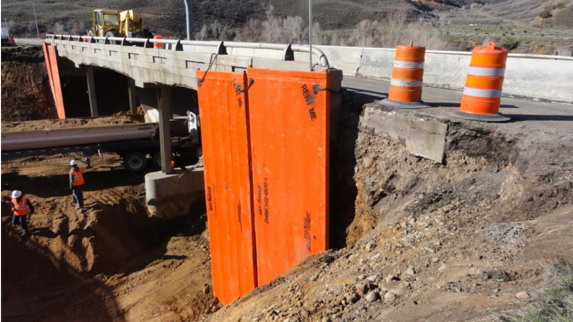
Figure 21. Photo. Shoring panels.
