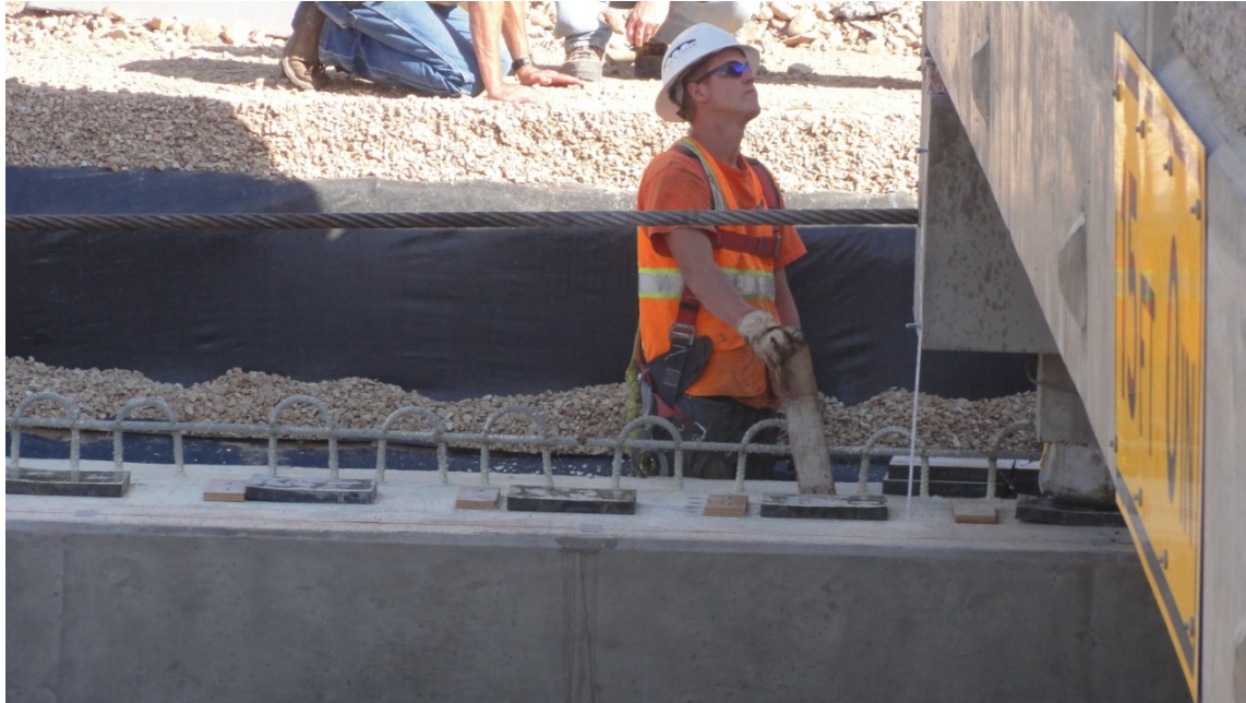
Figure 51. Photo. Bridge being slid across.
