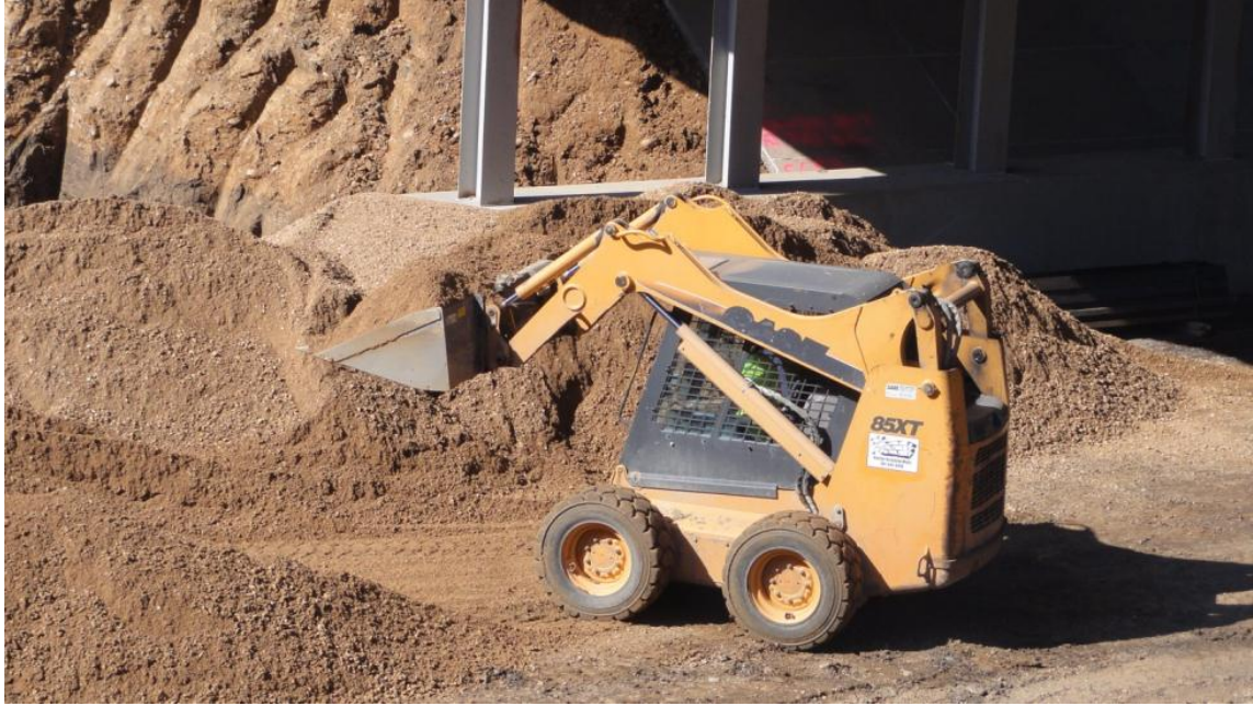
Figure 23. Photo. Soil being distributed across the site.
