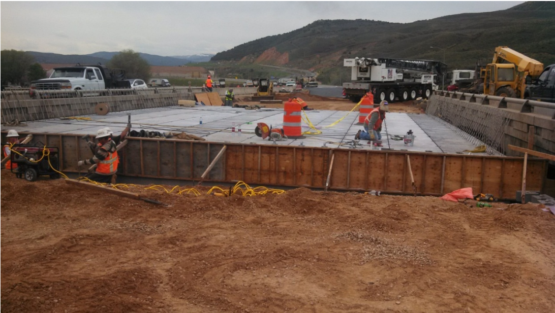
Figure 39. Photo. Bridge deck on the median bridge (courtesy: UDOT).
