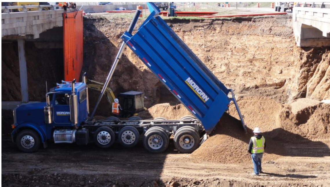
Figure 22. Photo. Dump trucks unloading soil for backfill purposes.
