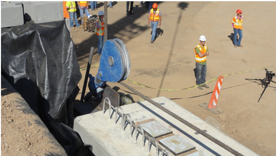
Figure 46. Photo. Snatch block connecting to the cable.
