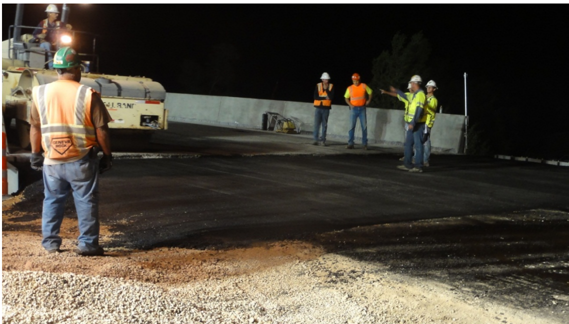
Figure 54. Photo. Overnight paving in the eastbound direction.
