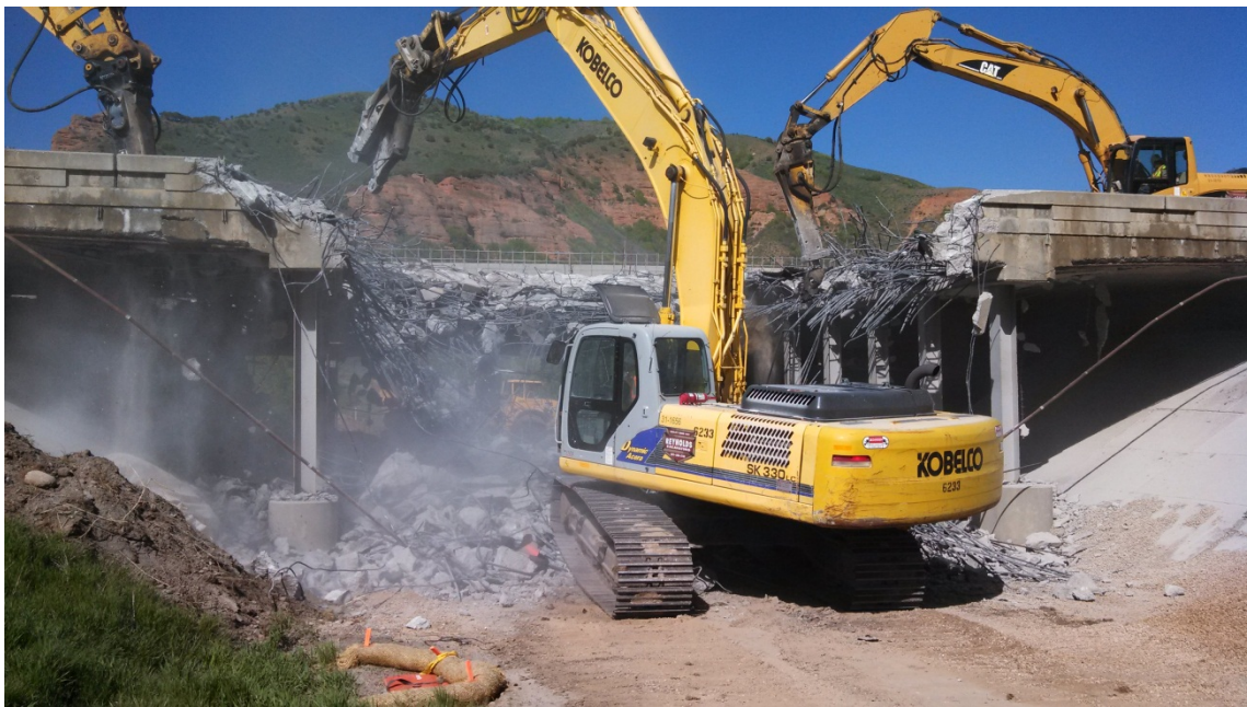
Figure 35. Photo. Eastbound bridge being demolished (courtesy: UDOT).
