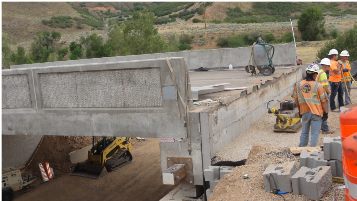
Figure 52. Photo. Bridge slide completed.
