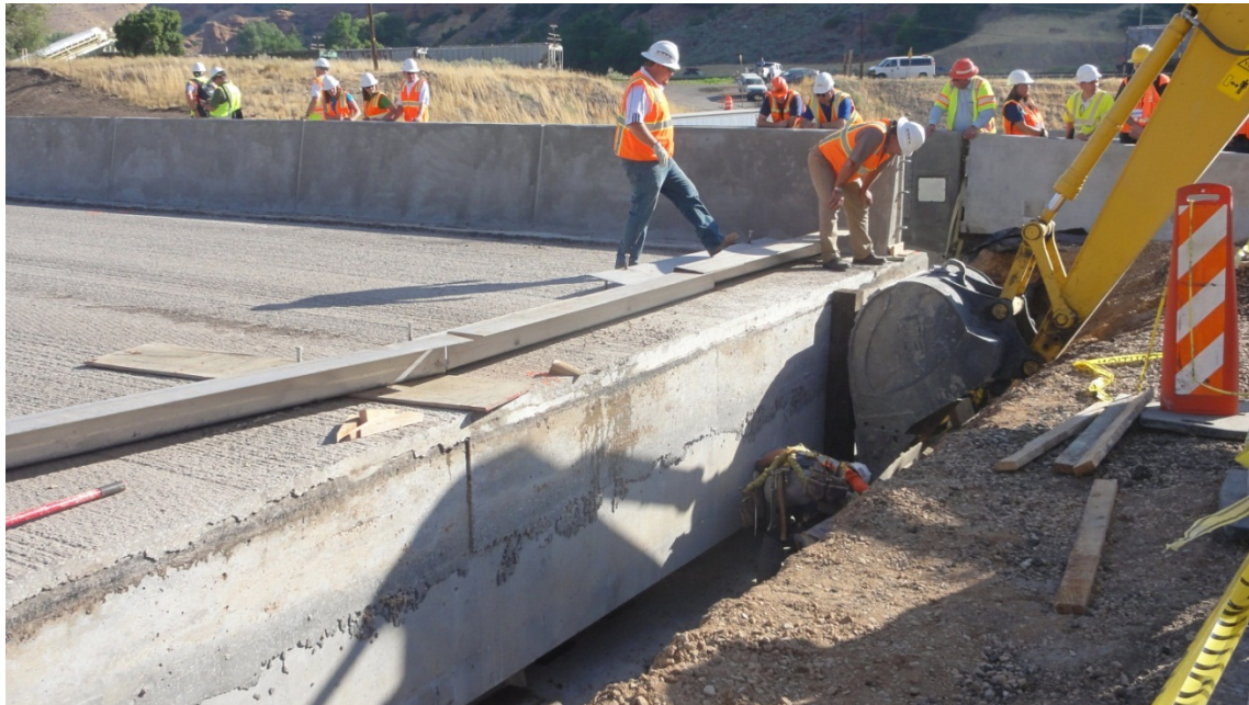
Figure 50. Photo. Backhoe used to control the horizontal slide in one direction.
