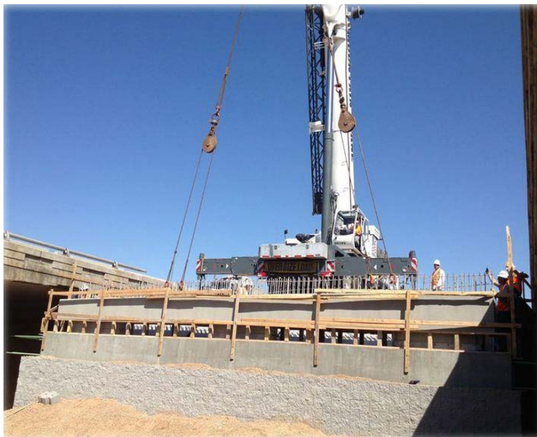
Figure 44. Photo. Bridge diaphragm being placed at the center median (courtesy: UDOT).
