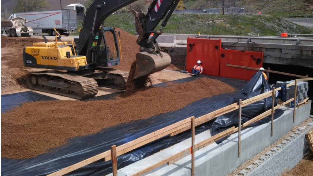
Figure 36. Photo. Geotextile-wrapped layers placed above the bridge footing (courtesy: UDOT).
