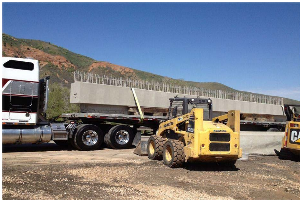
Figure 40. Photo. Bridge diaphragm being delivered to the site (courtesy: UDOT).
