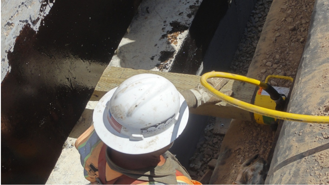
Figure 49. Photo. Push/pull jacks employed for better horizontal control during the slide.
