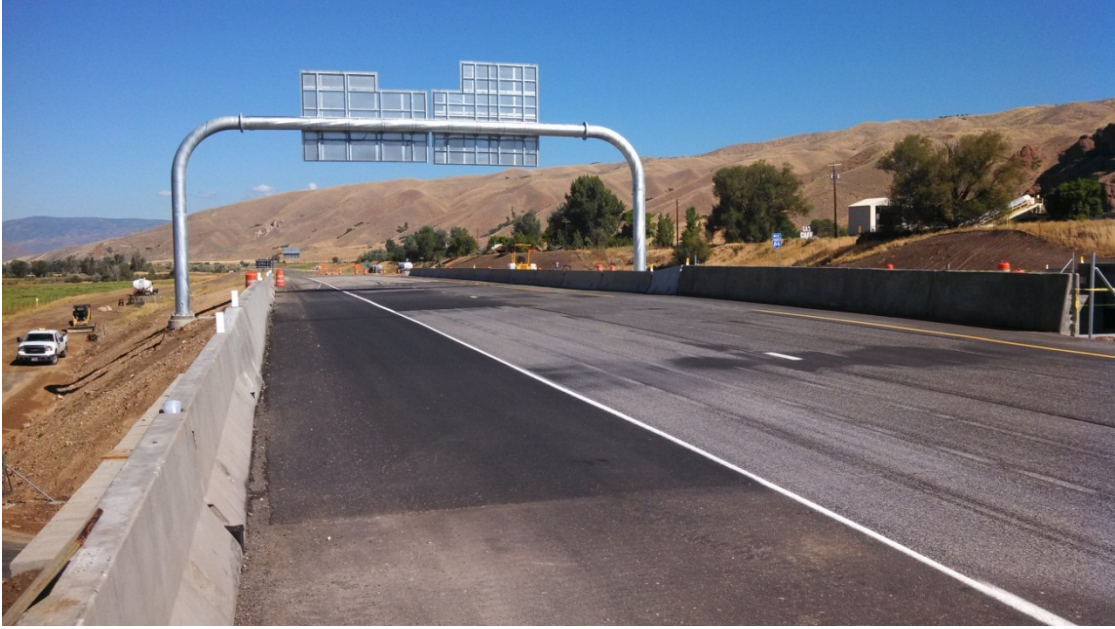
Figure 55. Photo. Eastbound bridge opened to traffic (courtesy: UDOT).
