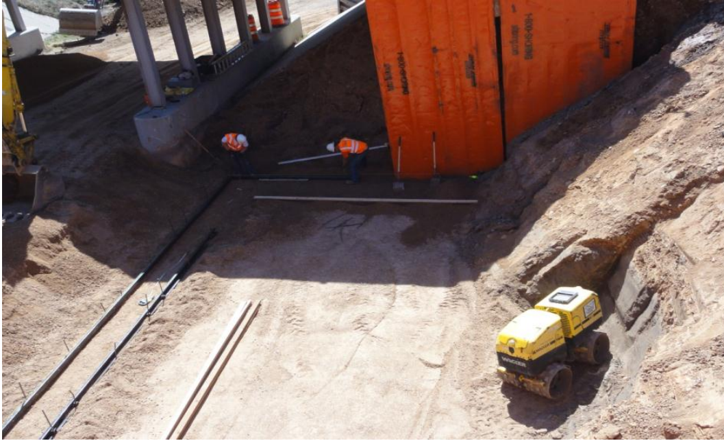
Figure 25. Photo. Formwork for leveling pads.
