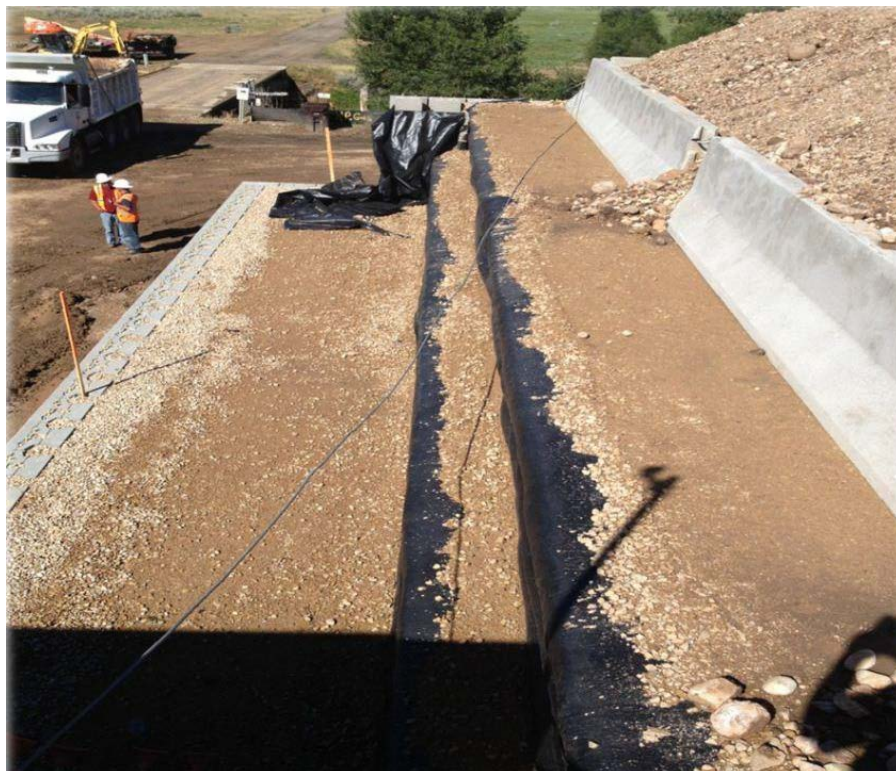
Figure 15. Photo. Surcharge placed on the eastbound bridge (courtesy: UDOT).
