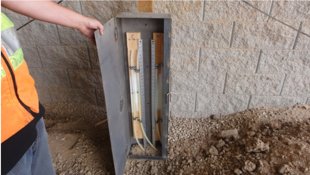
Figure 16. Photo. Settlement platforms.
