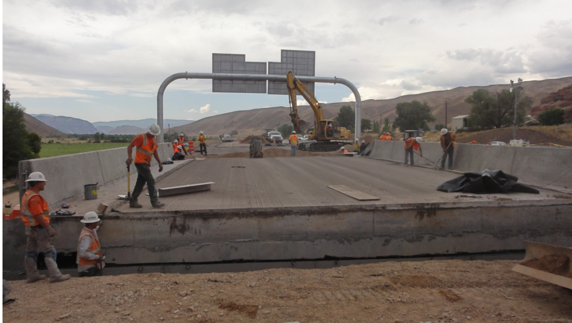
Figure 53. Photo. Eastbound bridge slid into final location.
