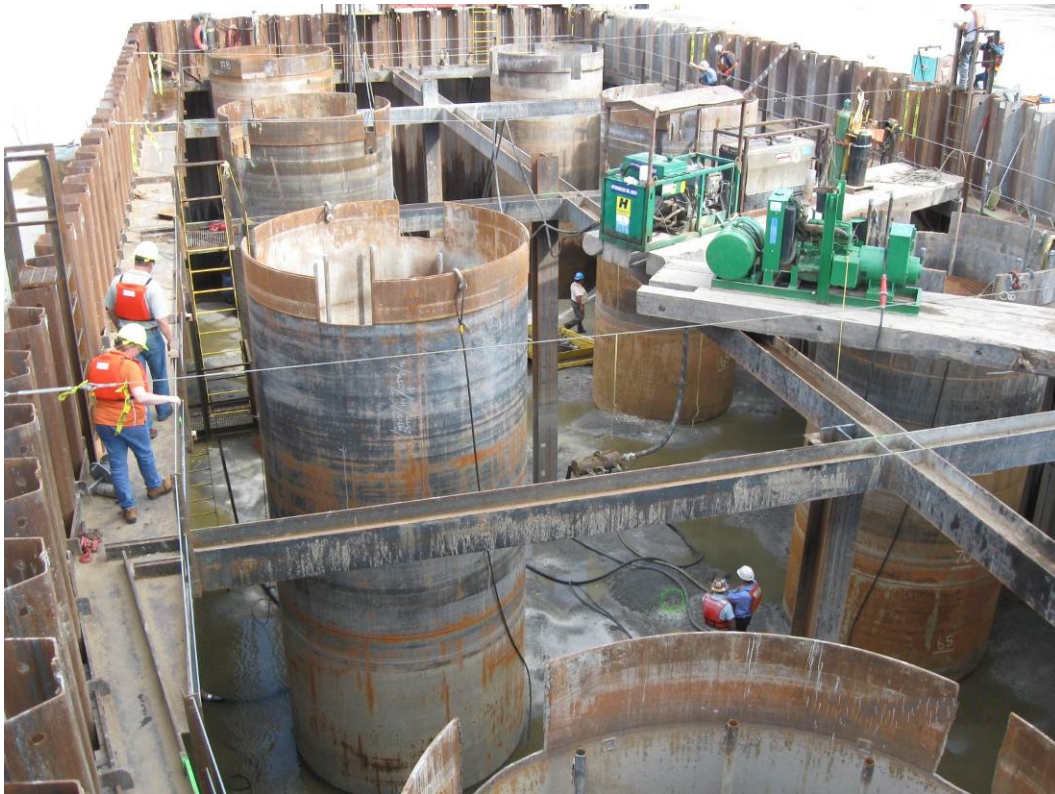
Figure 36. A dry cofferdam—October 2008.
