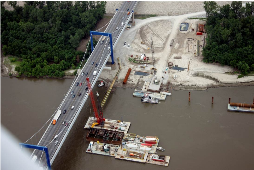
Figure 28. Aerial view of the cofferdam—August 2008.
