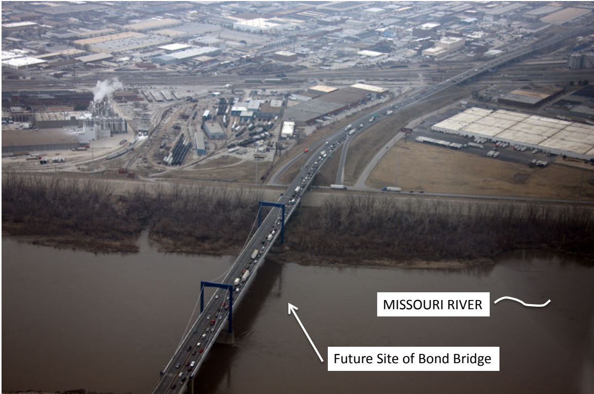
Figure 13. Four-lane Paseo Bridge crossing the Missouri River—March 2008.
