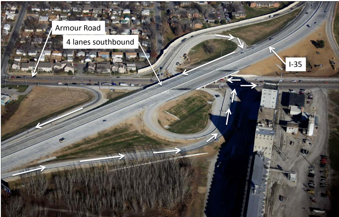
Figure 20. Armour Road interchange—January 2011.
