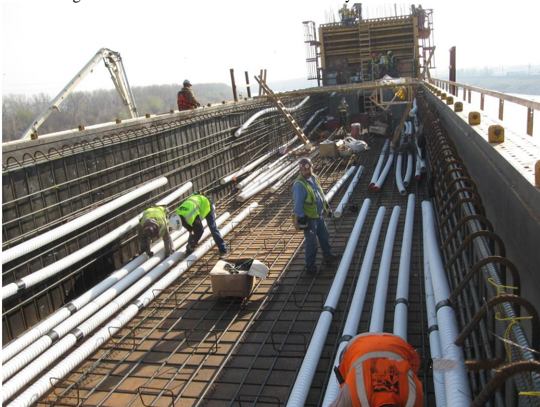
Figure 44. Placing reinforcement in the roadway strut—April 2009.
