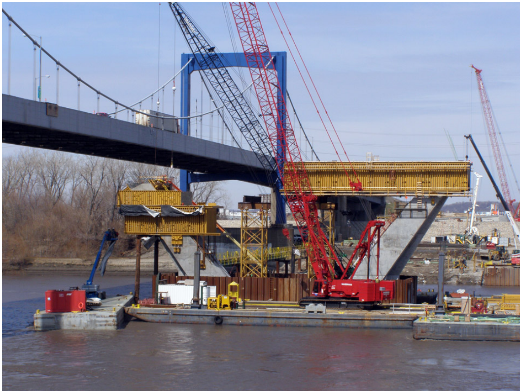
Figure 42. Constructing the roadway strut—March 2009.
