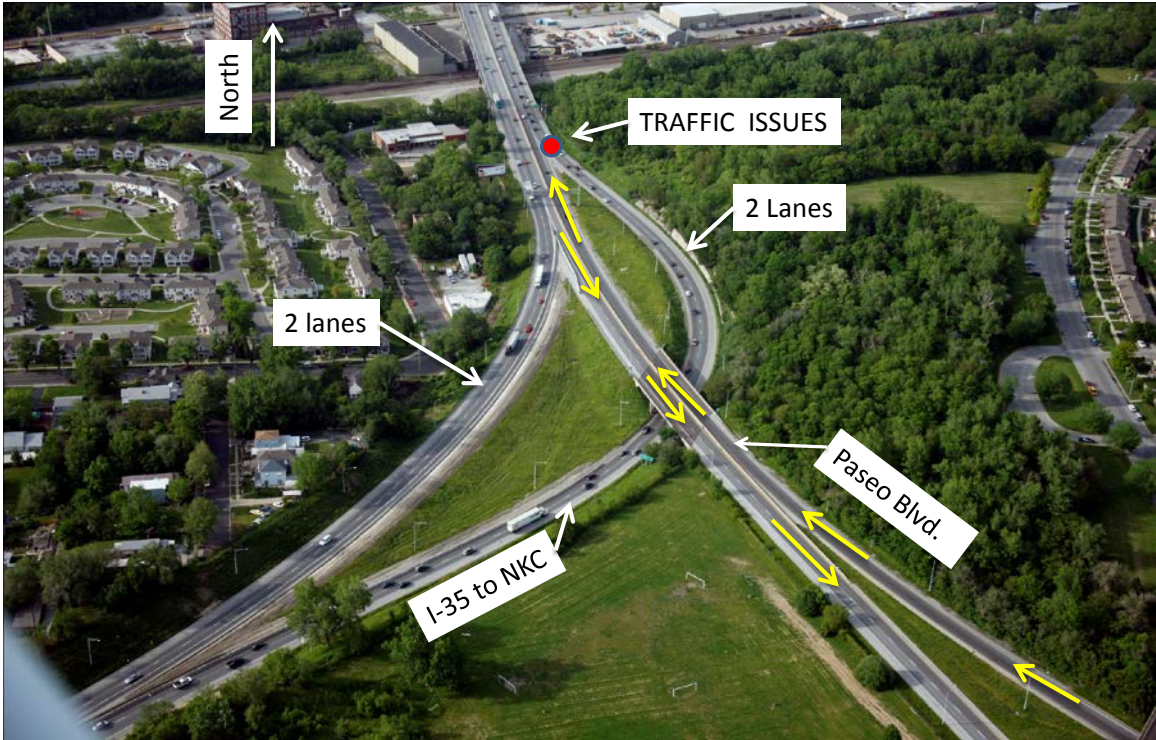
Figure 9. South end of project—March 2008.
