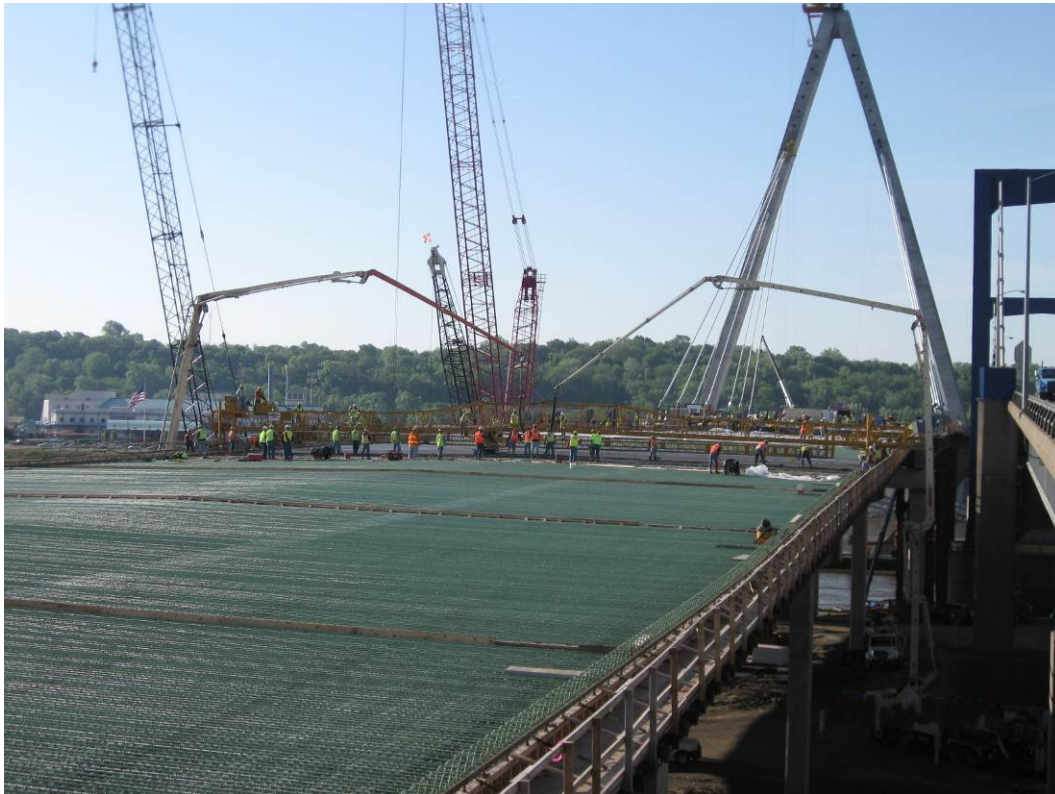
Figure 54. Bridge deck placement—April 2010.
