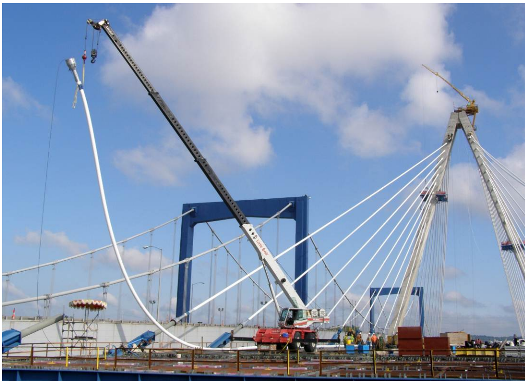
Figure 56. Final stay cable installed—August 2010.
