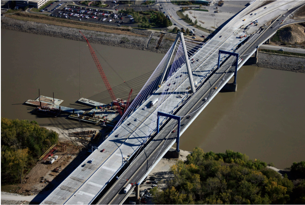
Figure 59. Christopher S. Bond Missouri River bridge—November 2010.
