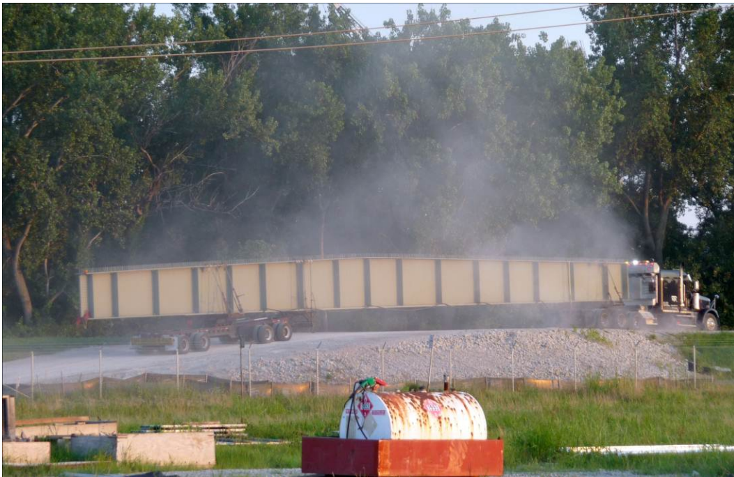
Figure 46. First bridge floor beam, 133 ft long and 66,500 pounds—August 2009.
