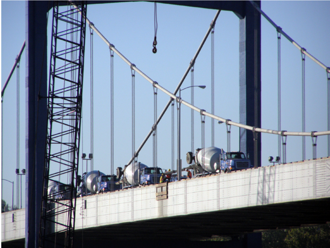
Figure 33. Delivery of concrete from the deck of the Paseo Bridge—October 2008.
