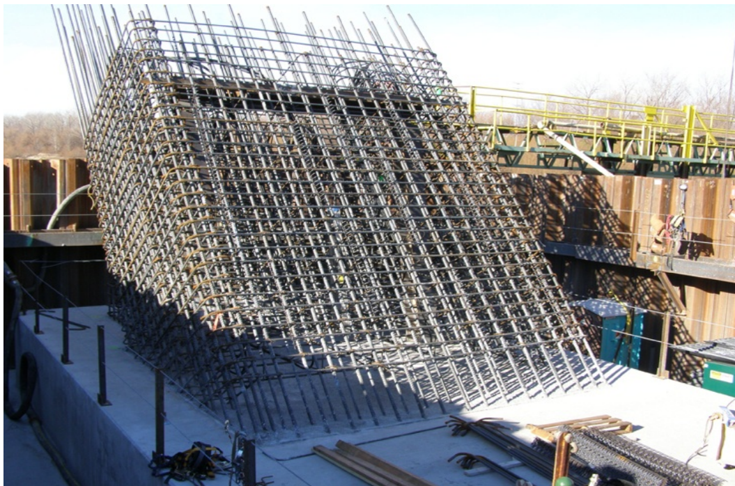
Figure 40. Rebar in place for the first concrete lift—November 2008.
