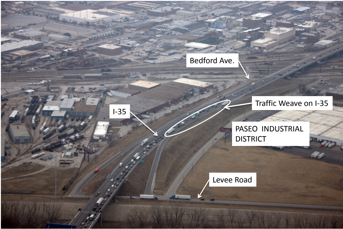
Figure 15. Levee Road crossing—March 2008.
