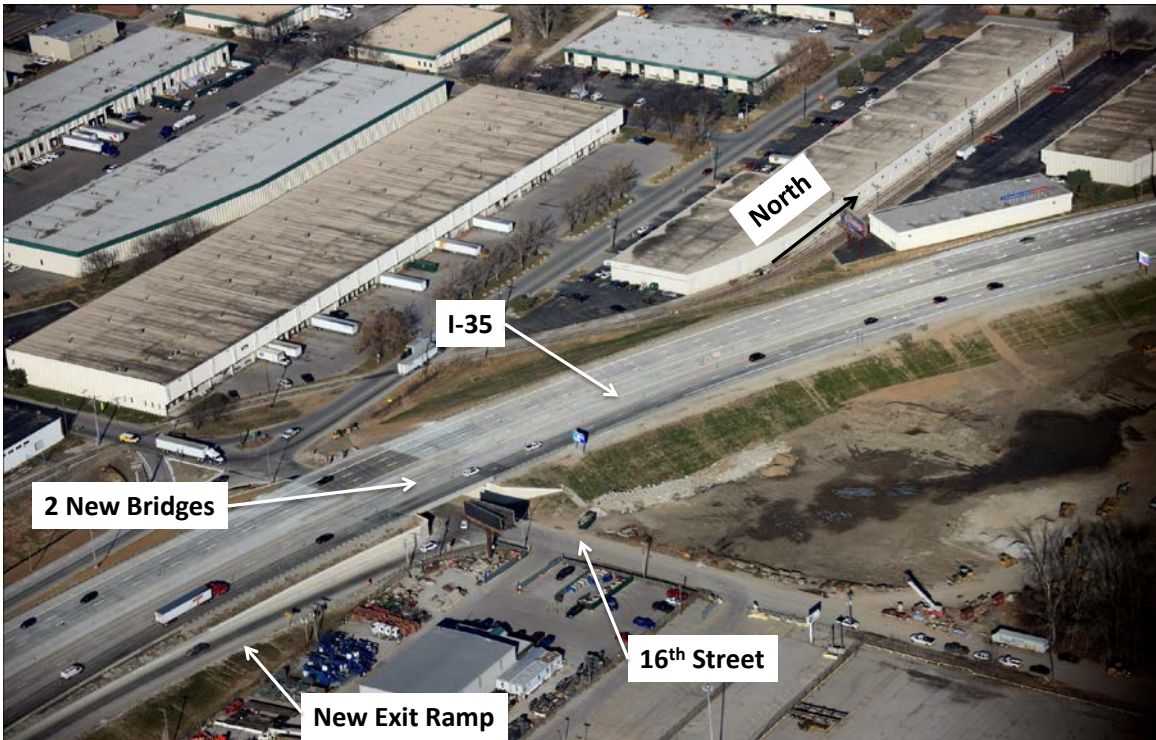
Figure 18. 16th Street exit ramp—January 2011.
