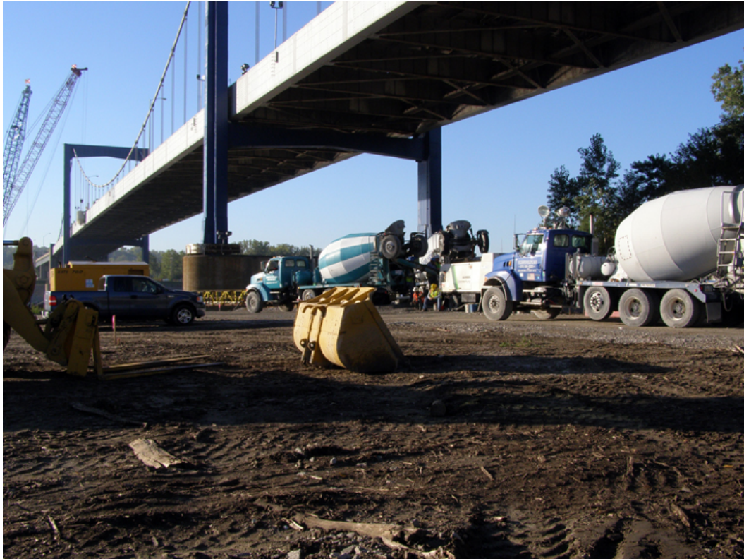
Figure 34. Delivery of concrete from below the deck of the Paseo Bridge—October 2008.
