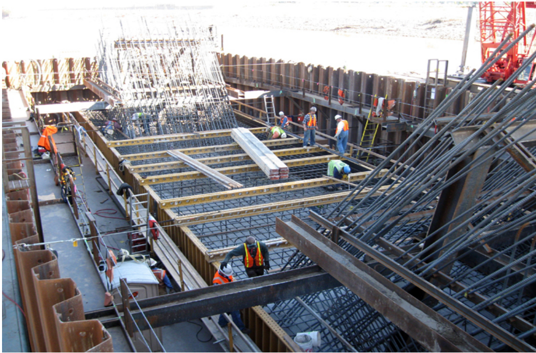
Figure 39. A total of 235 mi of rebar work—November 2008.
