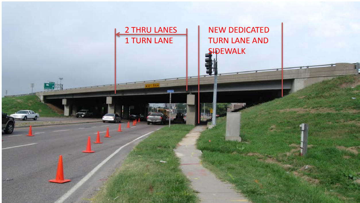
Figure 21. Armour Road and I-29/35—July 2008.
