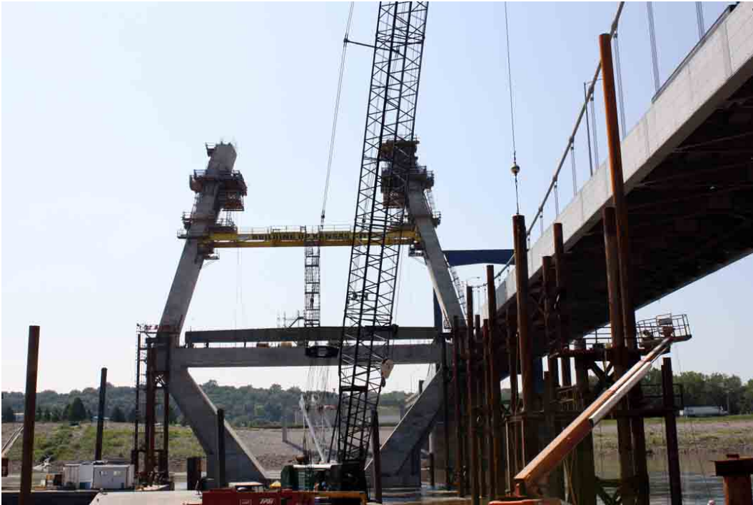
Figure 48. Temporary falsework supports the backspan roadway girders—August 2009.
