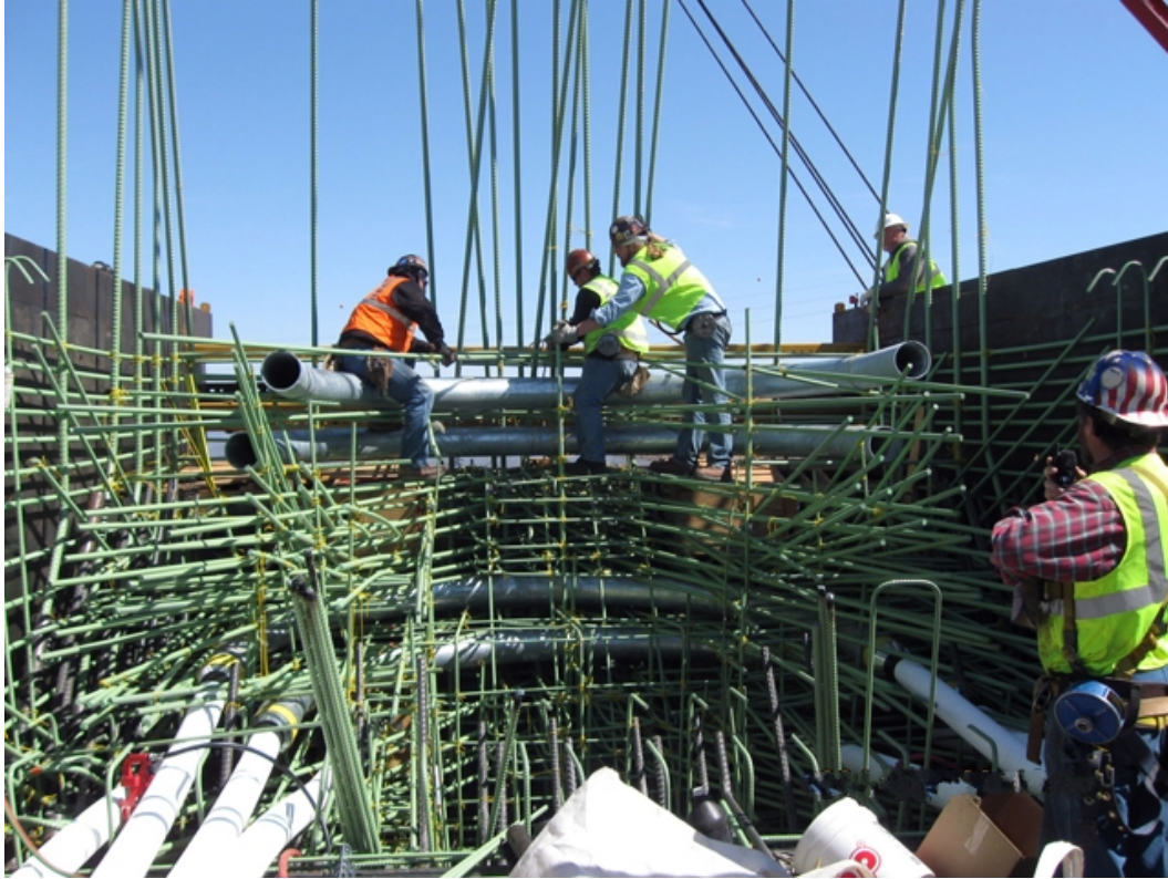
Figure 43. Inside the knuckle of the roadway strut—March 2009.
