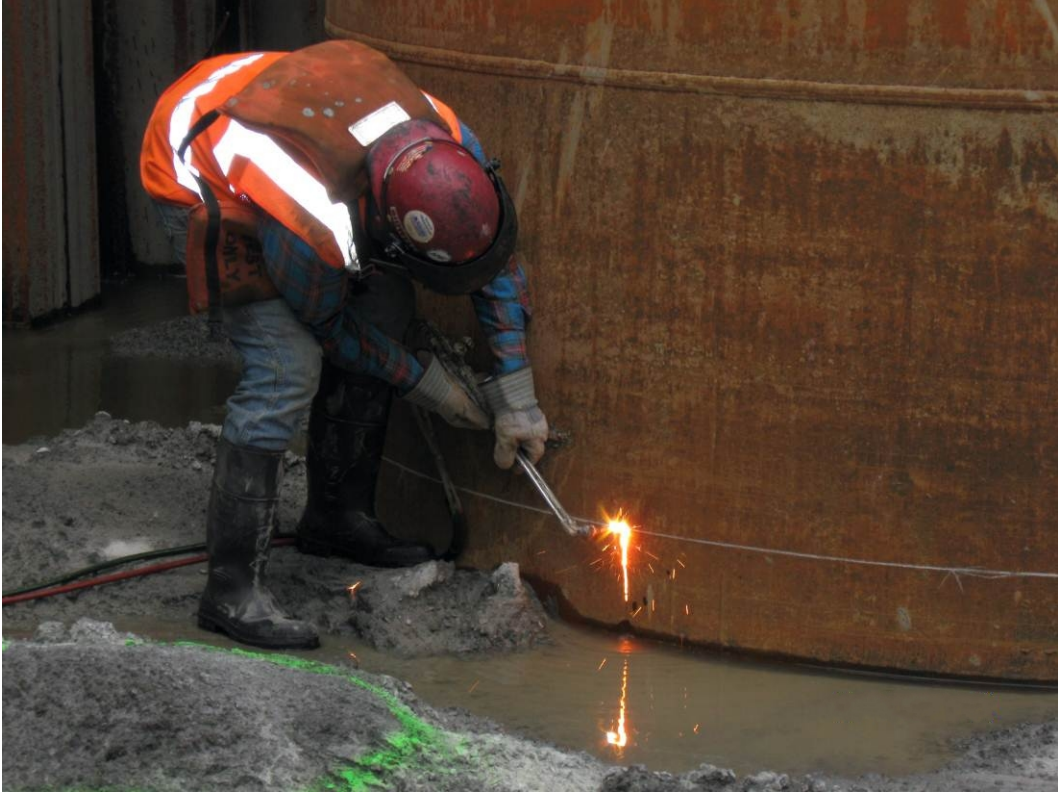
Figure 37. Cutting away the casings—October 2008.
