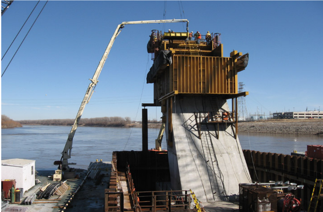
Figure 41. Placing concrete for second lift of downstream pylon leg—November 2008.
