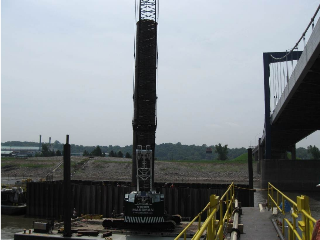
Figure 24. Lowering the permanent casing into the temporary casing—August 2008.
