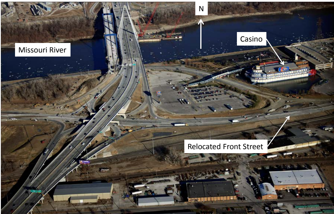
Figure 12. SPUI at Front Street—January 2011.
