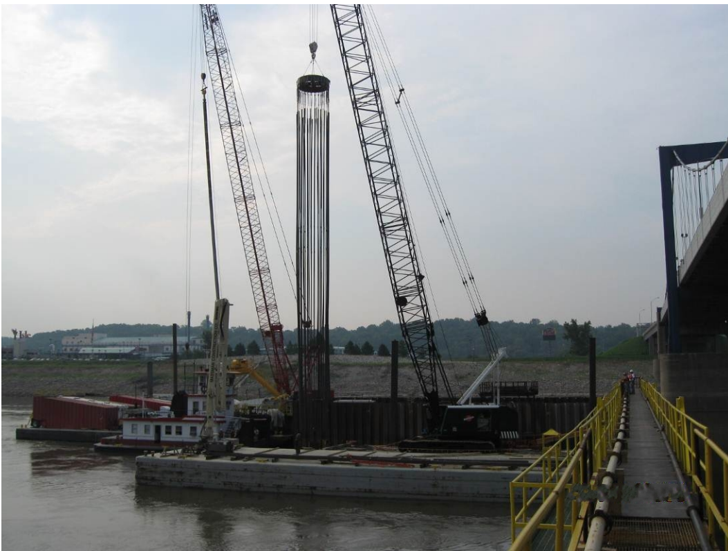
Figure 30. Swinging the rebar to the drilled shaft sleeve—August 2008.
