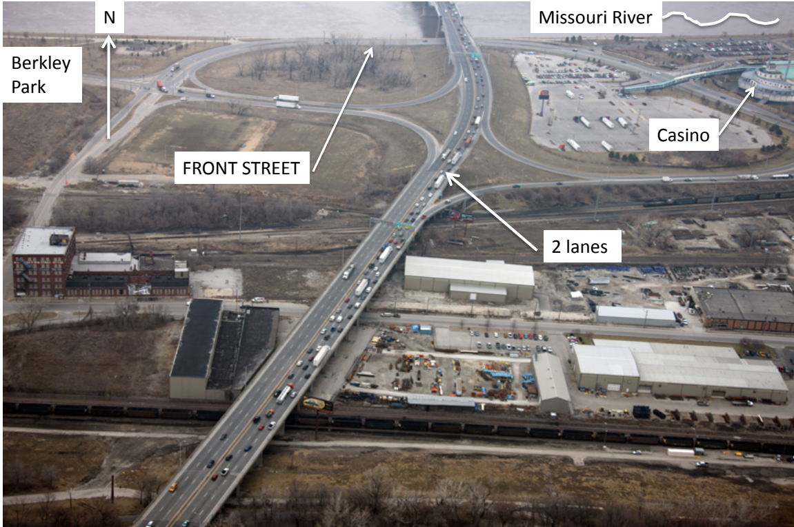
Figure 11. Front Street interchange—March 2008.
