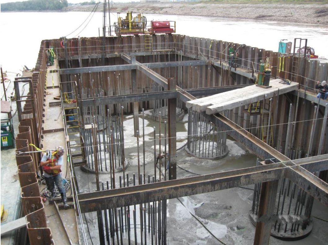
Figure 38. Removed casings—October 2008.
