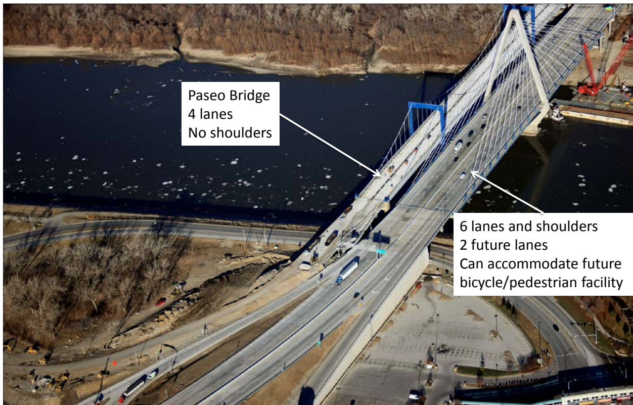
Figure 14. Six-lane Bond Bridge crossing the Missouri River—January 2011.
