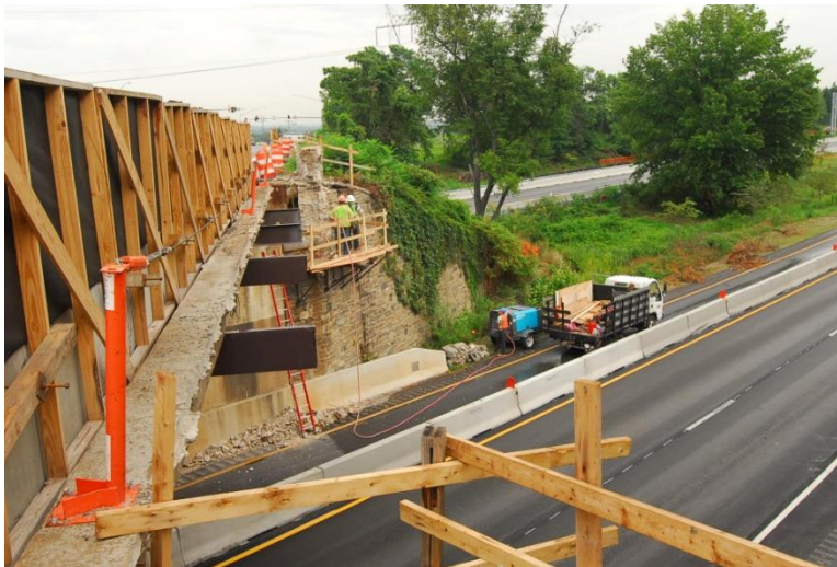
Figure 29. Existing superstructure with fascia beams removed.
