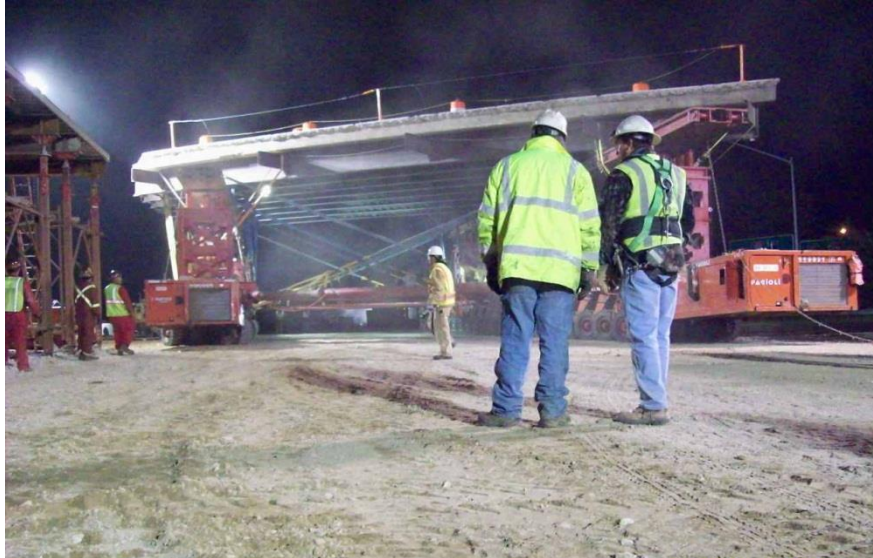
Figure 35. Old superstructure on MD 295 southbound being moved into place in the median.
