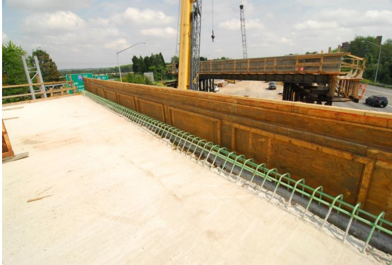
Figure 30. Reinforcement and formwork for parapet construction.
