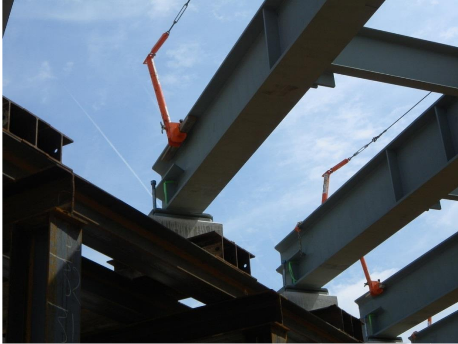
Figure 15. View of anchor bolts.
