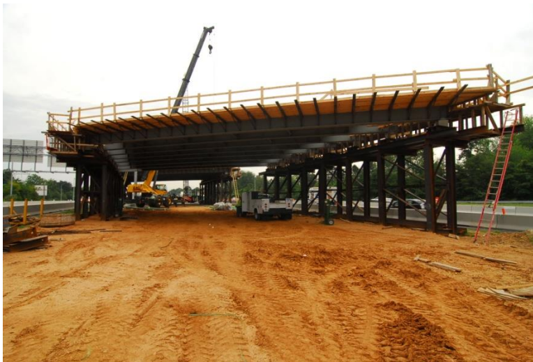
Figure 21. Progress on fabrication of new superstructures.
