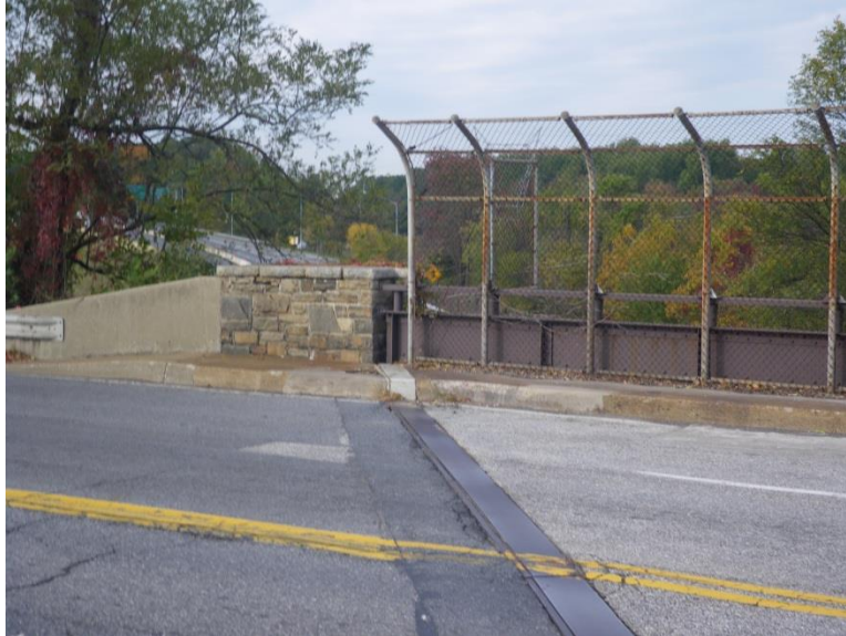
Figure 11. Old structure, showing sidewalks and severe skew.
