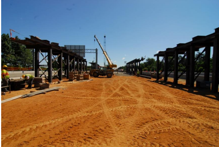
Figure 20. Median with temporary steel supports.
