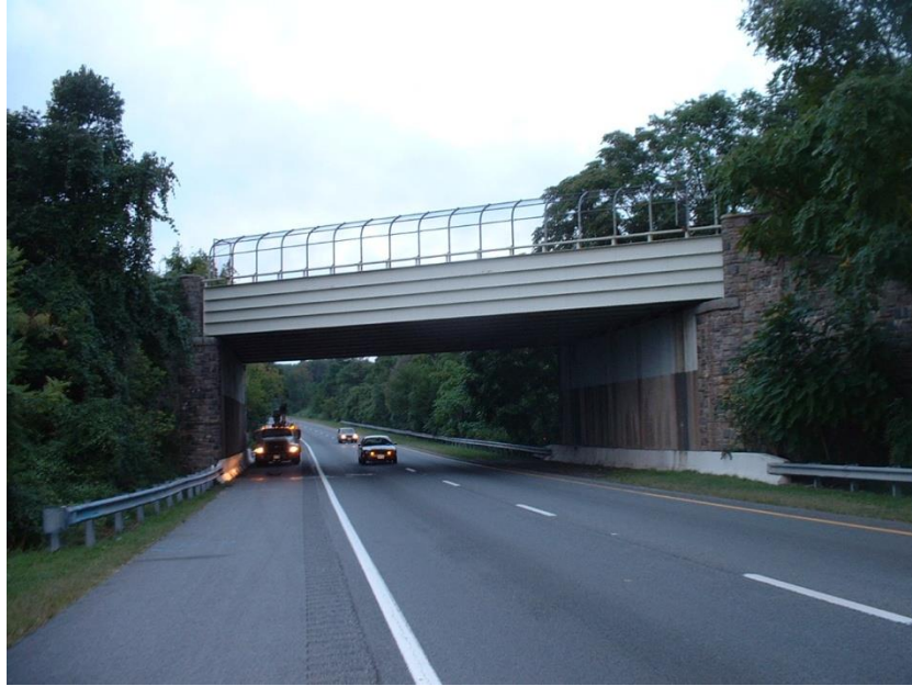
Figure 4. Elevation of Bridge No. 02014 (northbound).
