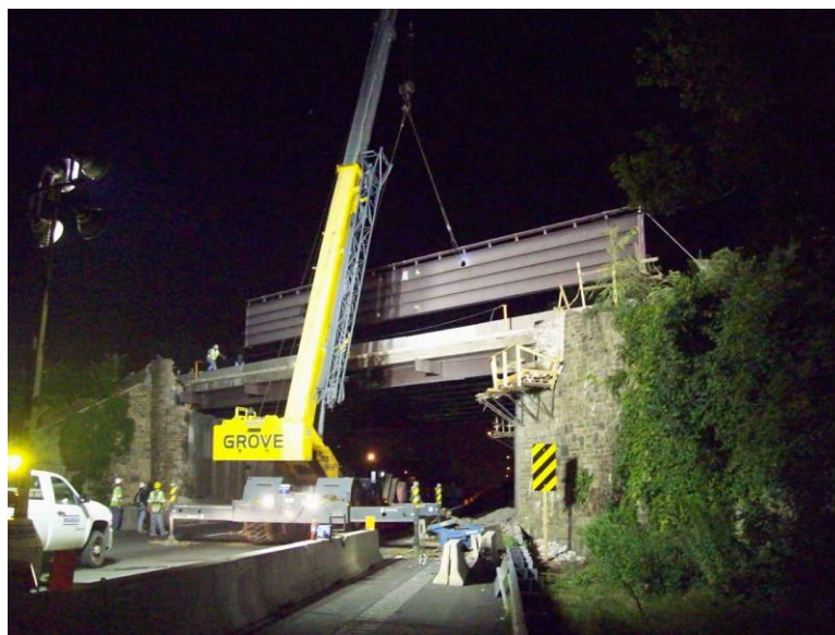
Figure 25. Removal of fascia beam.
