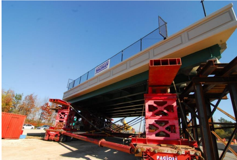
Figure 18. SPMT supporting completed superstructure for bridge over MD 295 northbound.
