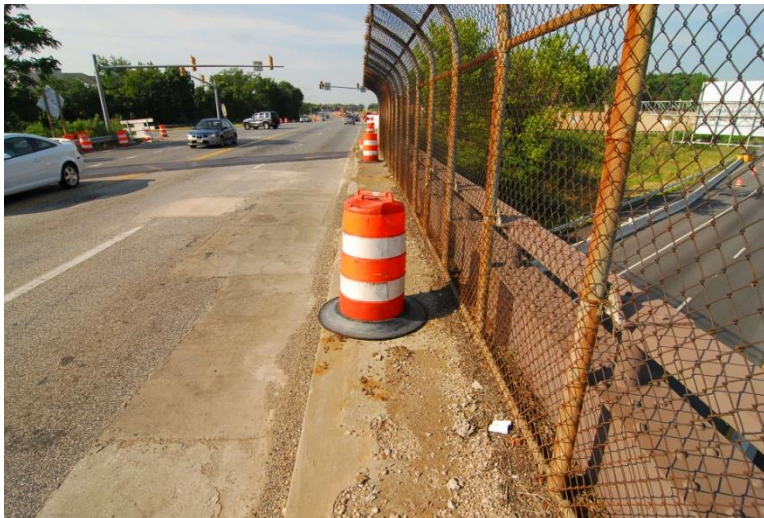
Figure 23. Existing superstructure with sidewalk, fence, and fascia beam.
