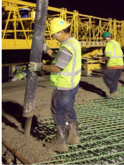
Figure 28. Deck concrete placement.
