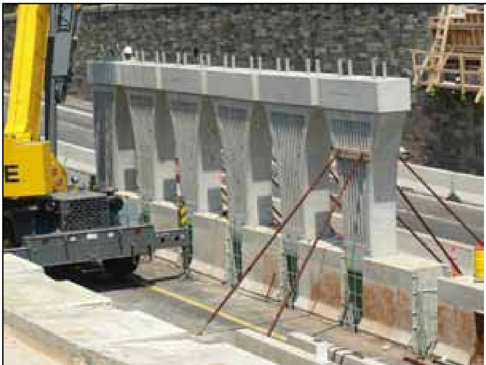
Figure 8. Installation of precast pier units.
