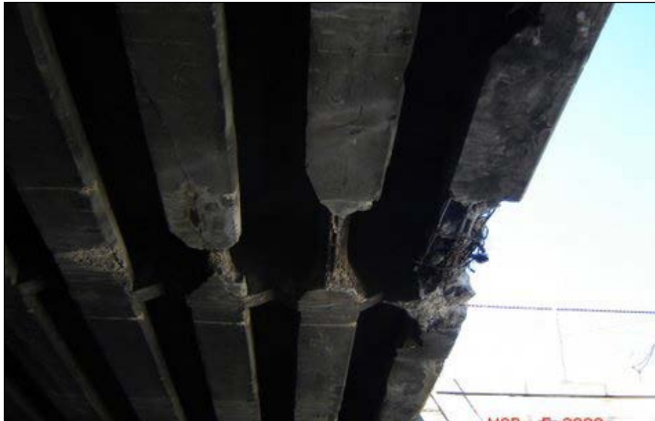
Figure 4. Closeup of damage to the bridge beams.
