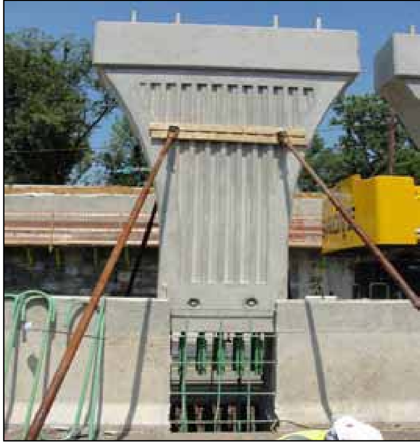
Figure 11. Connection between footing and precast pier units.
