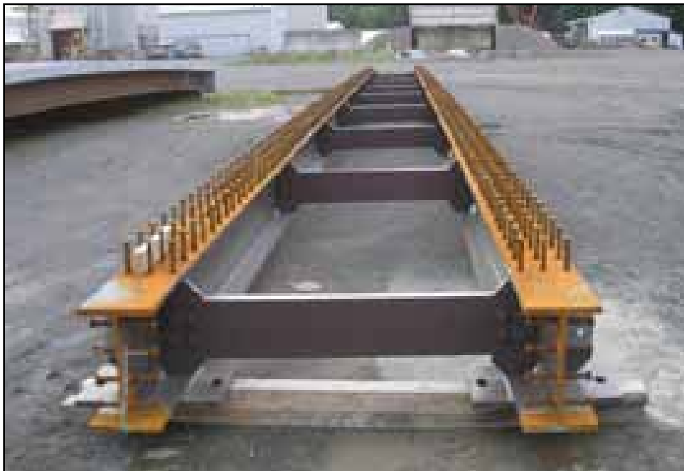
Figure 14. Steel assembly for a precast superstructure unit.
