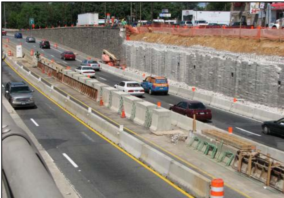
Figure 20. Traffic flow during construction of cast-in-place footing for the pier.
