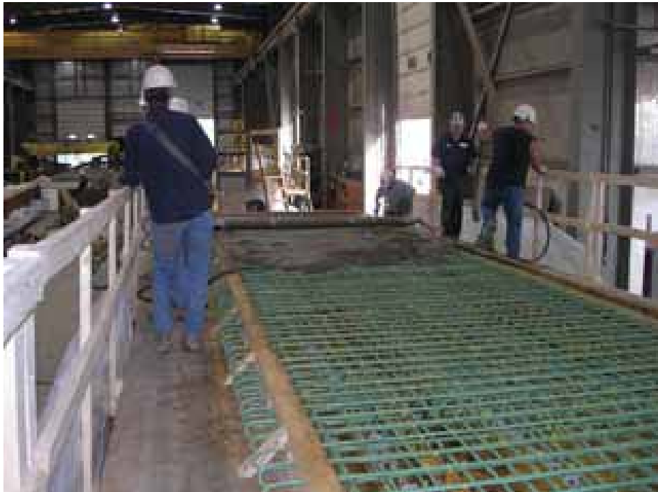
Figure 16. Steel reinforcement for a precast superstructure unit.
