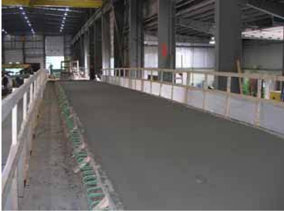
Figure 17. Finished precast superstructure unit.
