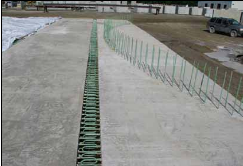
Figure 19. Adjacent superstructure units with connection reinforcement.
