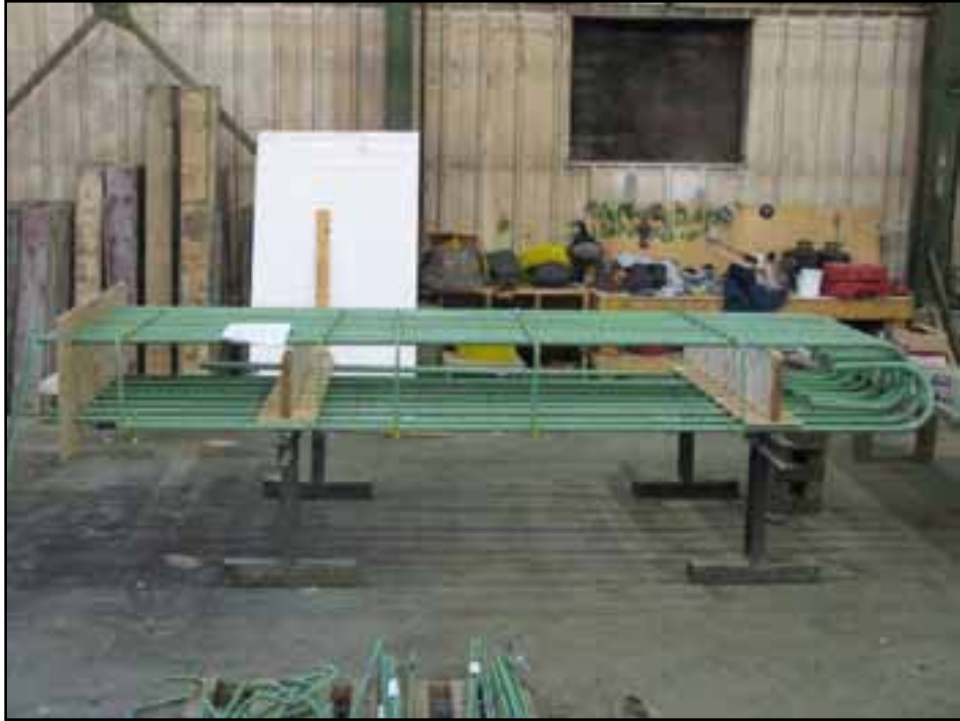
Figure 6. Reinforcement for precast pier unit.
