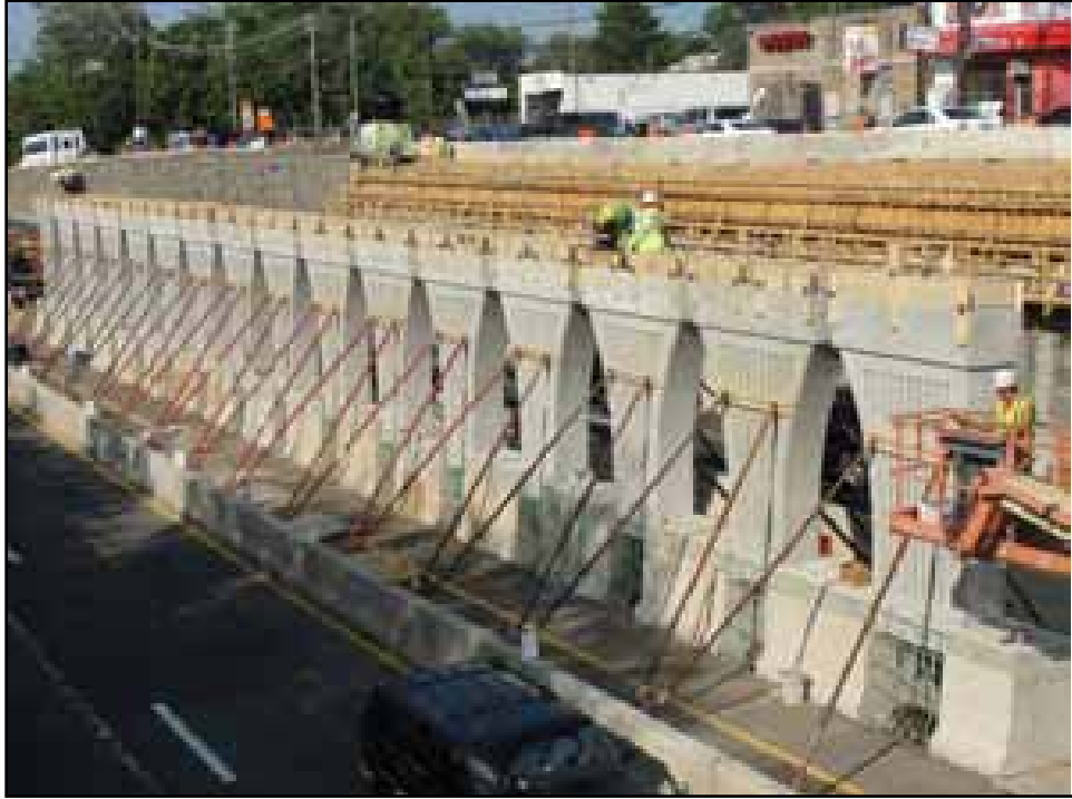
Figure 9. Pier installation (abutment reconstruction in background).
