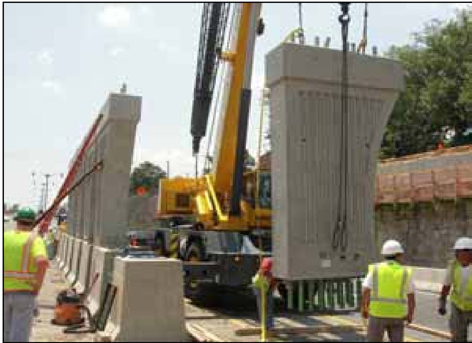
Figure 10. End pier installation.
