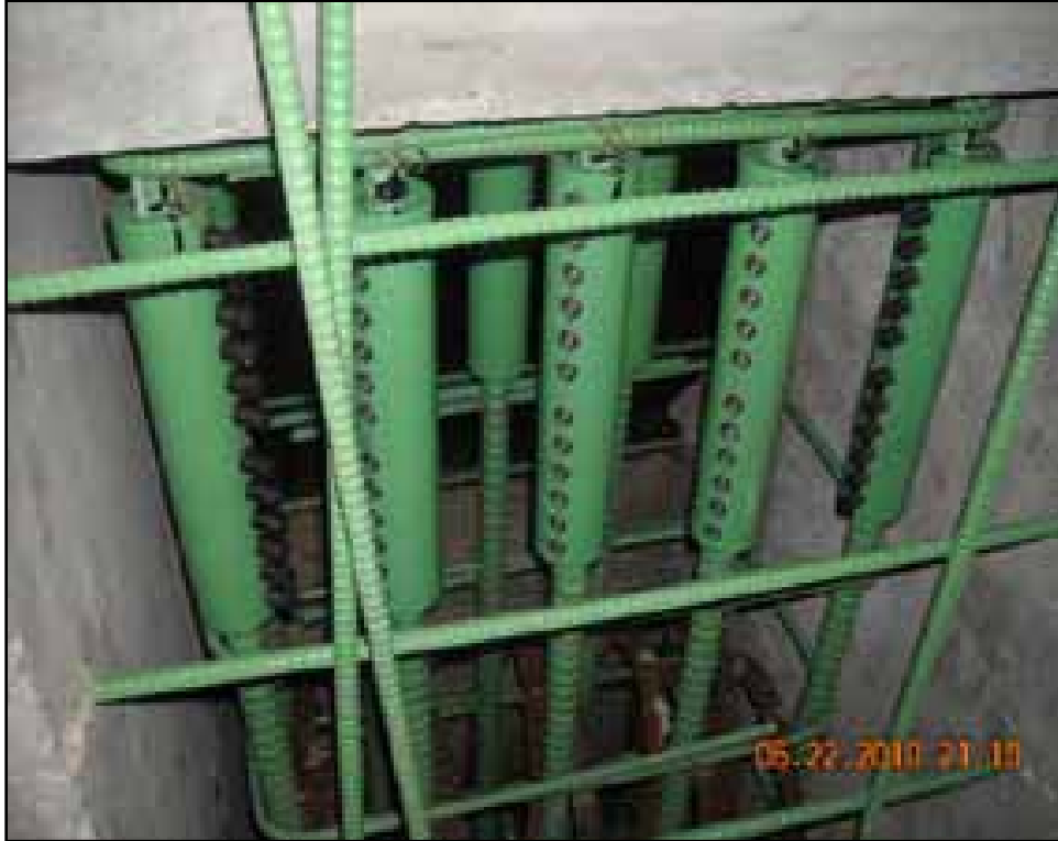
Figure 13. Closeup of the reinforcement steel couplers.
