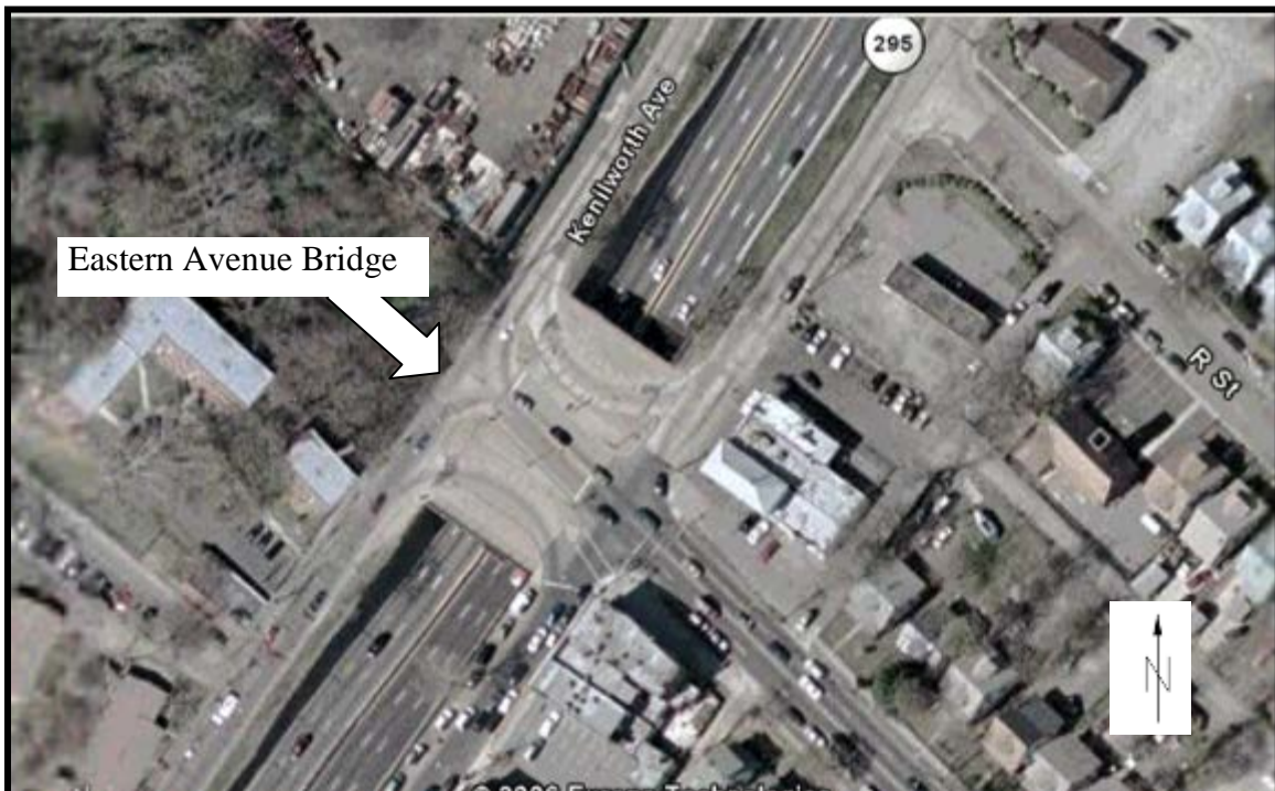
Figure 2. Preconstruction aerial photograph of Eastern Avenue bridge.
