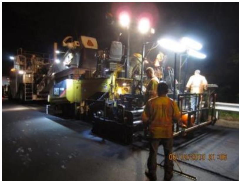
Figure 5. Photo. Paving of I-95.
