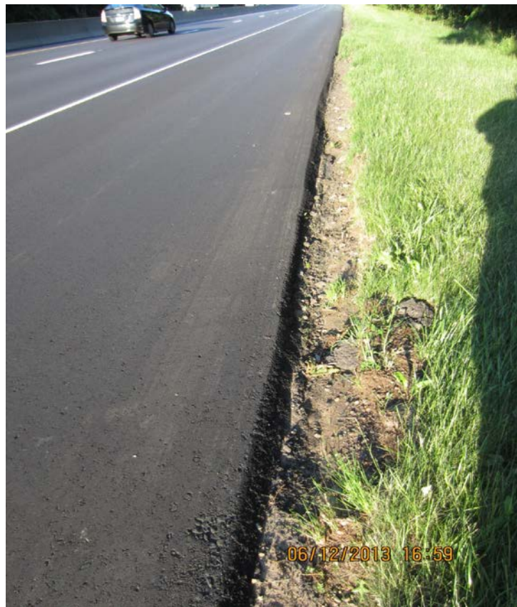
Figure 10. Photo. Formation of Safety Edge prior to backfilling along I-95.
