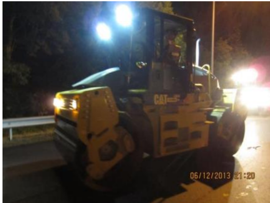
Figure 7. Photo. Compaction roller.
