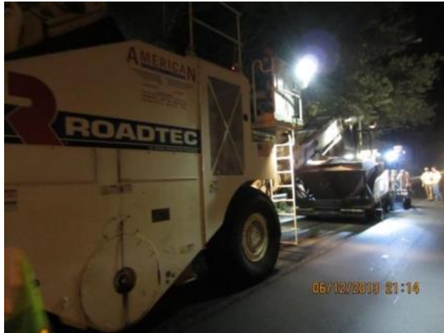
Figure 6. Photo. Roadtec material transfer device.
