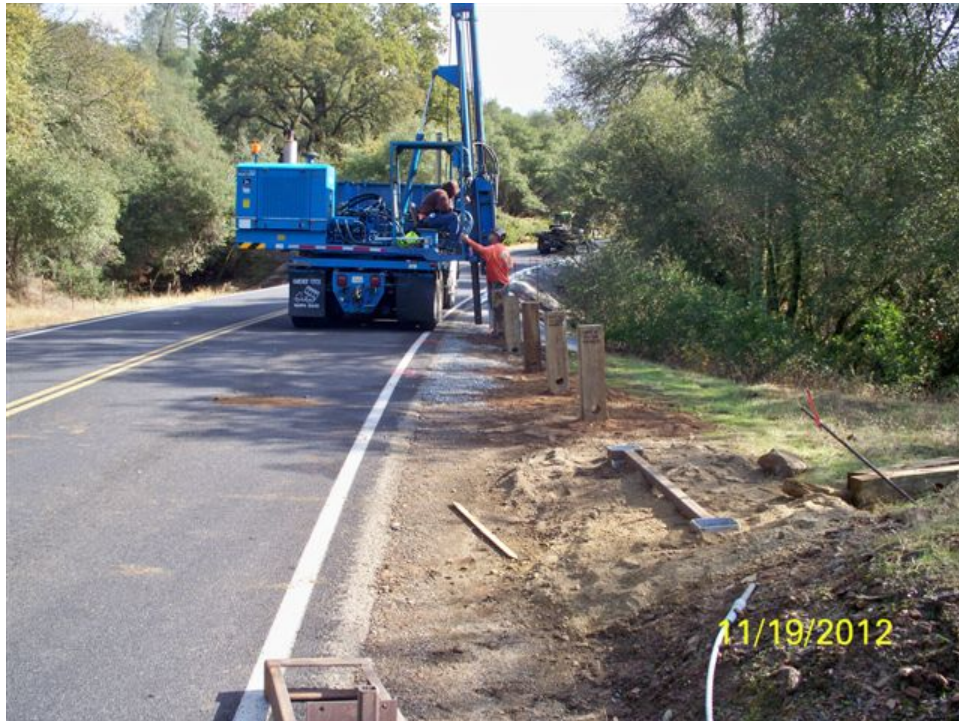
Figure 34. Driving the posts for the MBGR into the embankment material.
