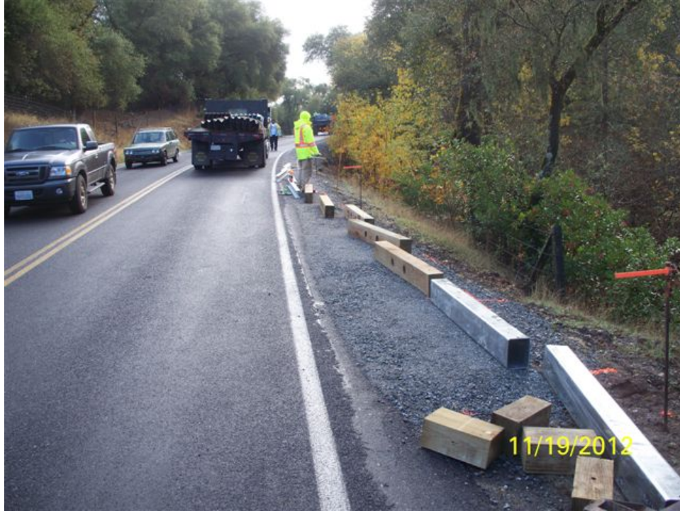
Figure 33. Preparation for installation of the MBGR.
