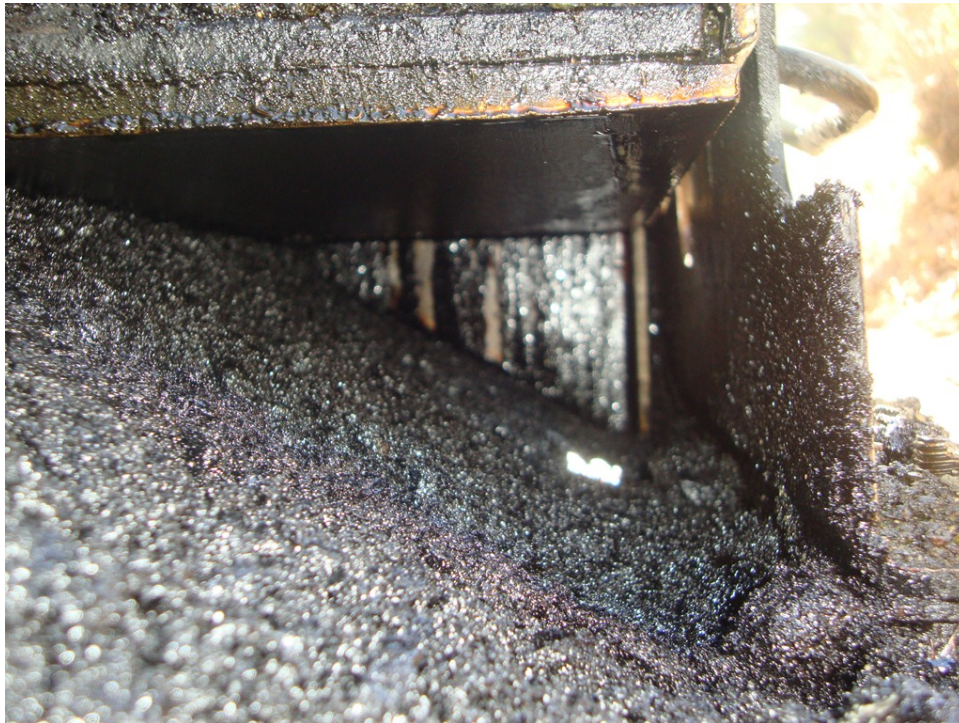
Figure 18. Safety Edge shoe of the Advantedge® device engaged onto the HMA to form the Safety Edge.
