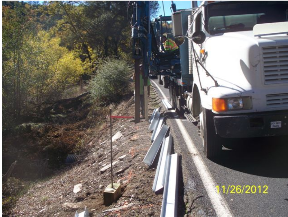
Figure 35. Driving the posts for the MBGR into the embankment material.
