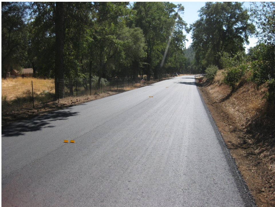
Figure 32. Finished roadway with Safety Edge.
