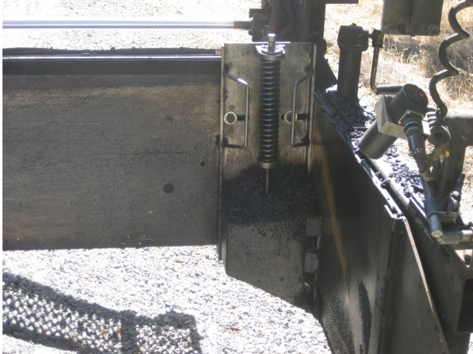
Figure 16. Advantedge® Safety Edge device installed on the paver screed.
