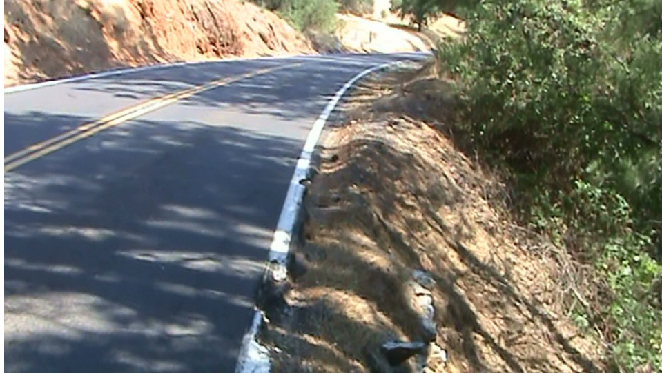
Figure 4. Typical narrow shoulders, acclivity on north (left) side of road, and declivity on south (right) side of Mountain Ranch Road.
