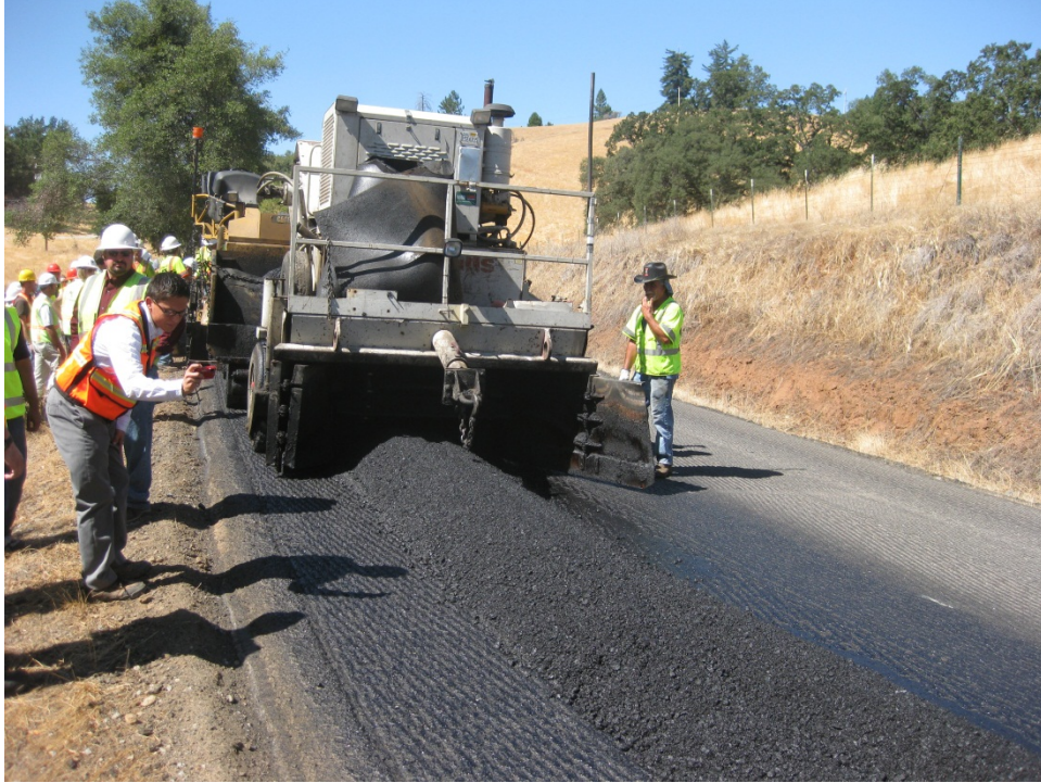
Figure 46. Participants observing the Safety Edge paving during the field trip.
