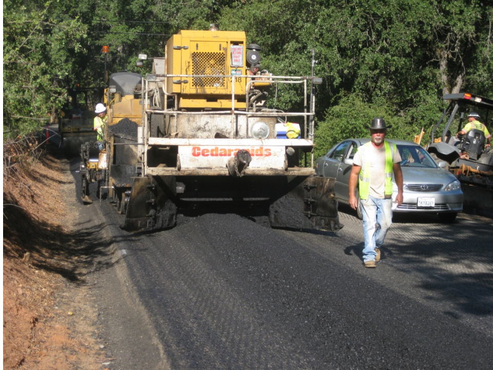
Figure 14. Paving Mountain Ranch Road.
