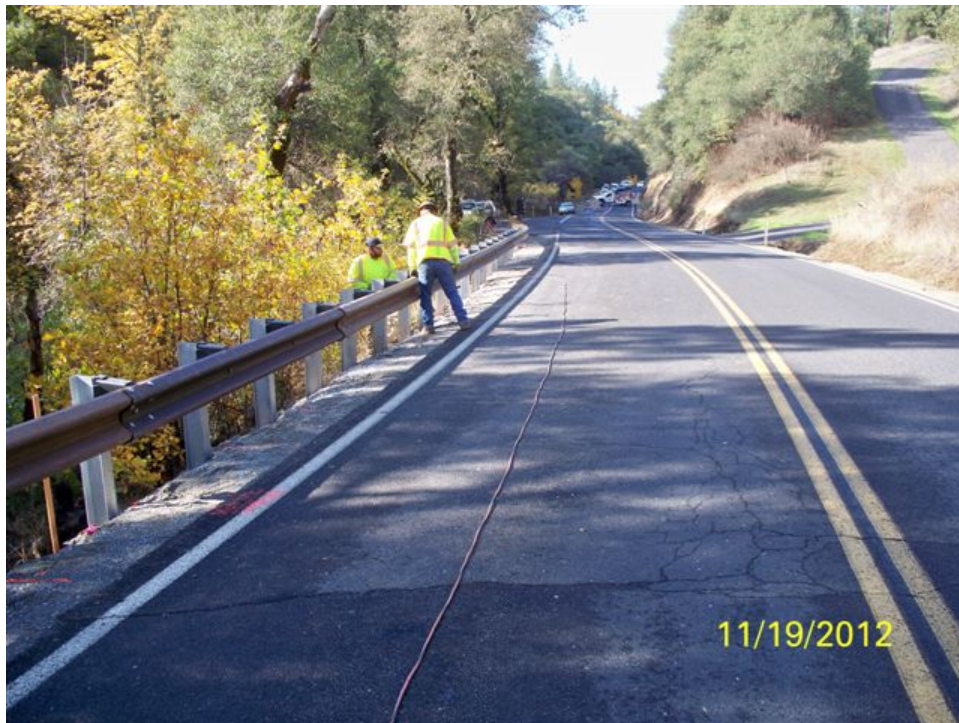
Figure 36. Installation of the MBGR.
