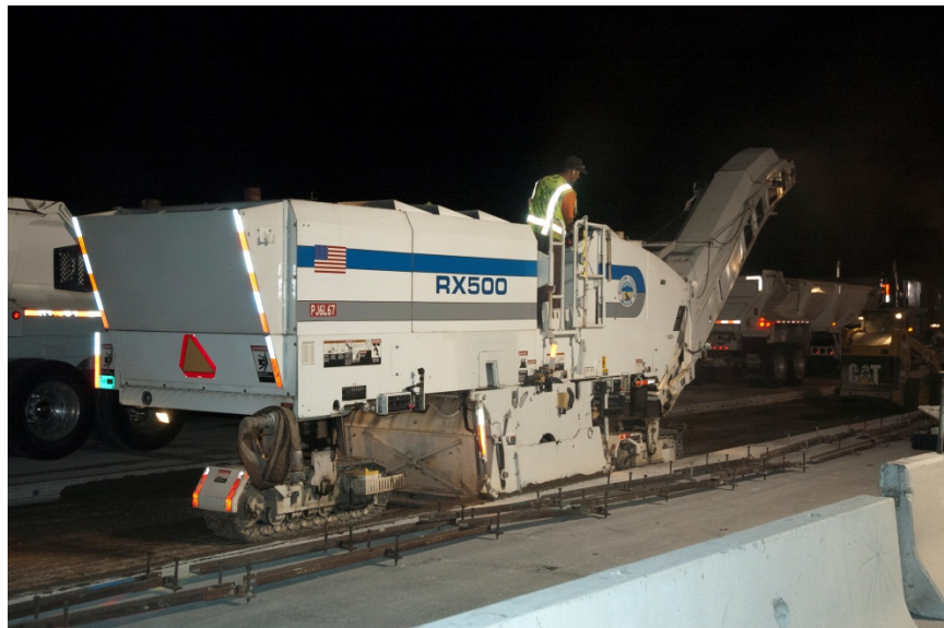
Figure 15. A milling machine is used to level the CTB as needed.
