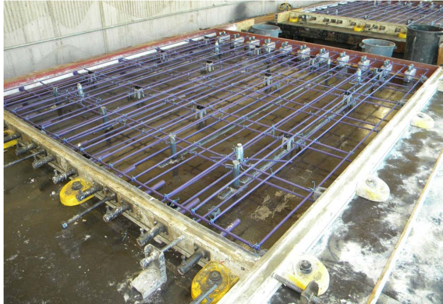
Figure 9. Epoxy-coated steel reinforcement is shown in a typical panel layout.
