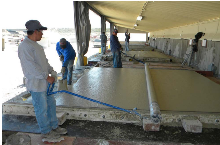
Figure 10. Workers use a roller-type screed to level the panels.
