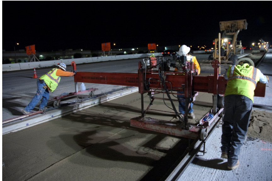
Figure 16. Workers use a track-mounted screed to level the base.
