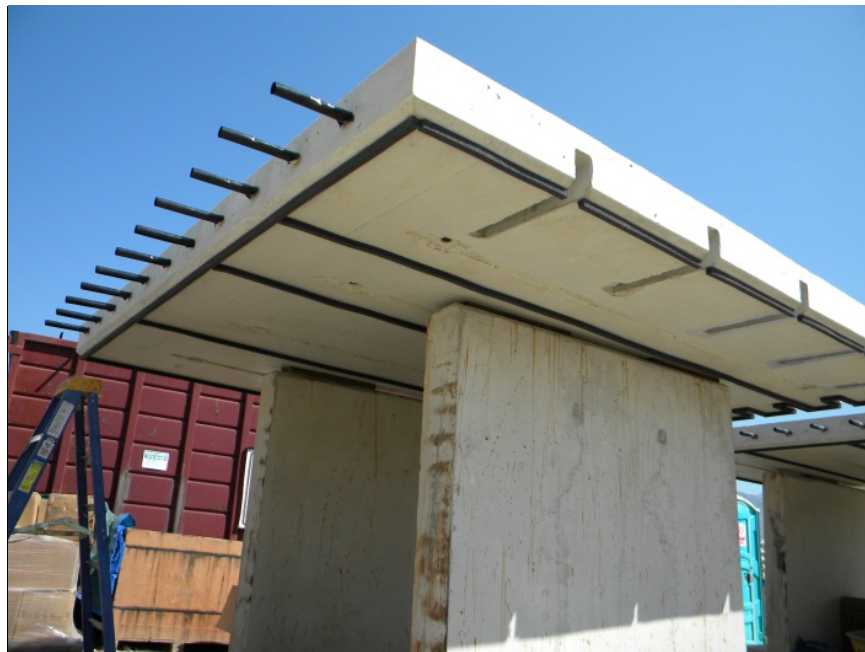
Figure 13. Underside of a panel. Note dowels bar and tie bar pockets.
