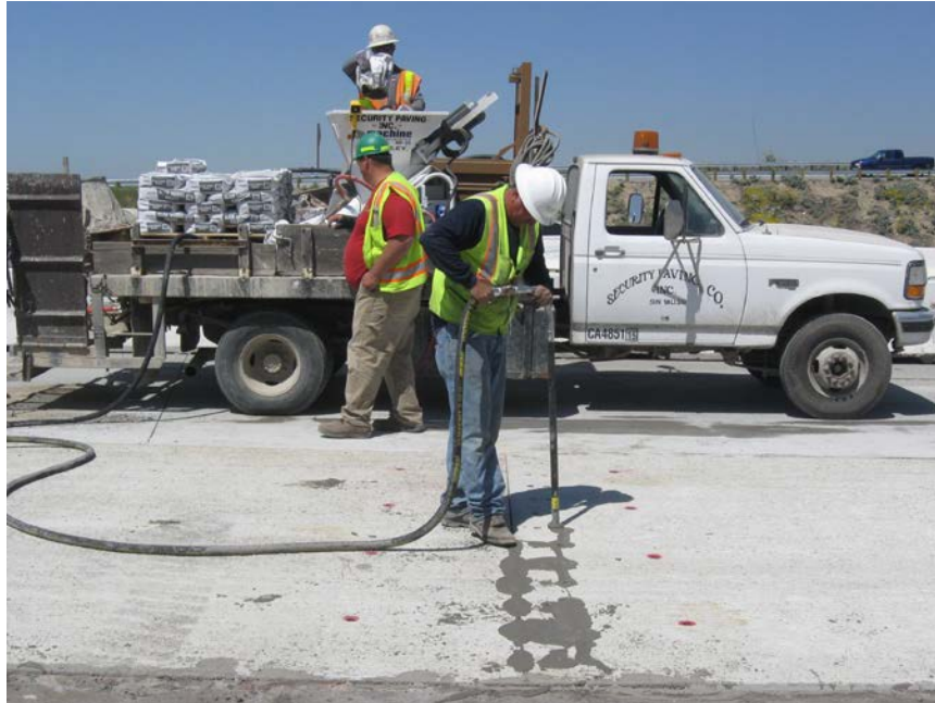
Figure 18. Grouting operation.
