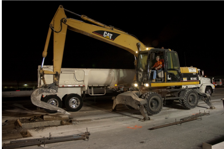
Figure 14. Existing panels were removed in manageable pieces.
