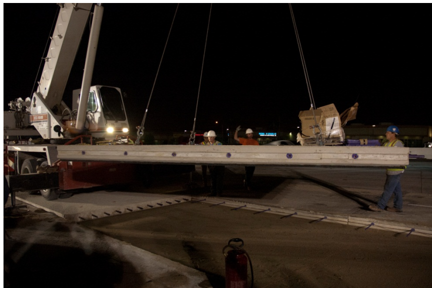
Figure 17. A panel is set in place.
