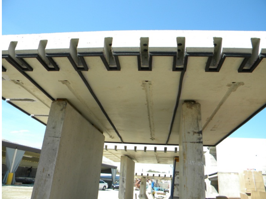
Figure 12. Underside of a panel. Note the gaskets, dowel pockets, and grooves for the bedding grout.
