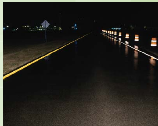
All-Weather Pavement Markings
