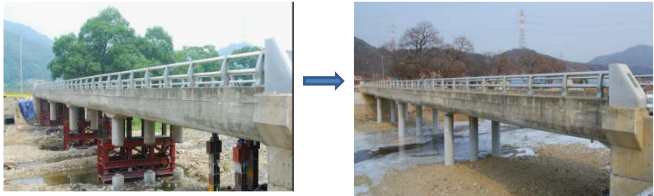
Figure 5: Retrofit of In-Service Bridges
