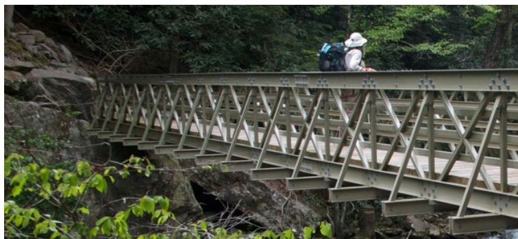
Rock Creek Bridge on the Cumberland Trail, Tennessee
