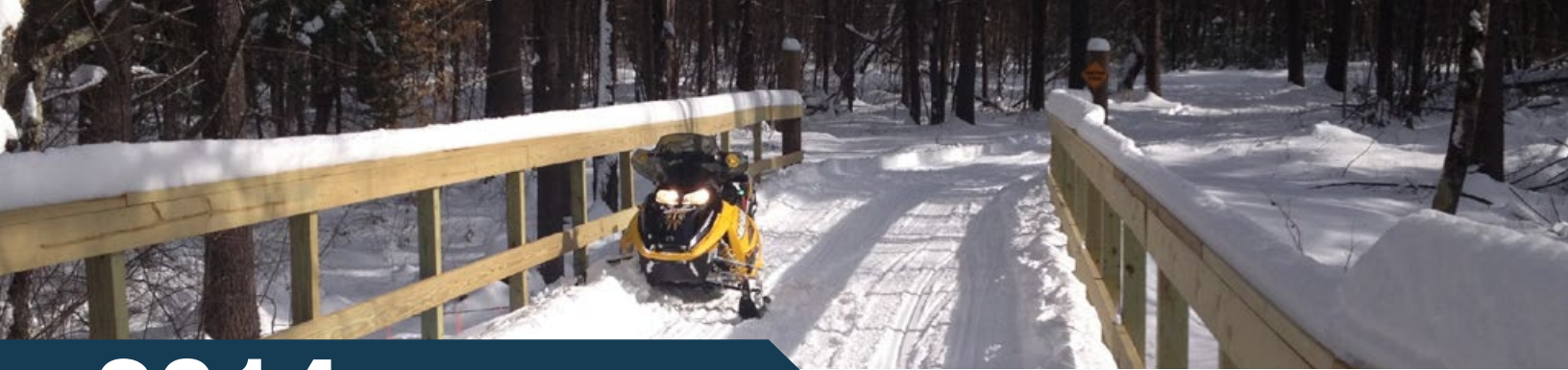
Fred W. Jones Memorial Bridge, Madison, New Hampshire
