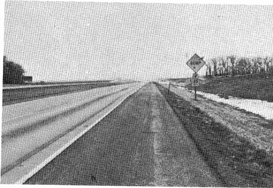
Figure 5.54. Swell Caused by Frost Heave.
