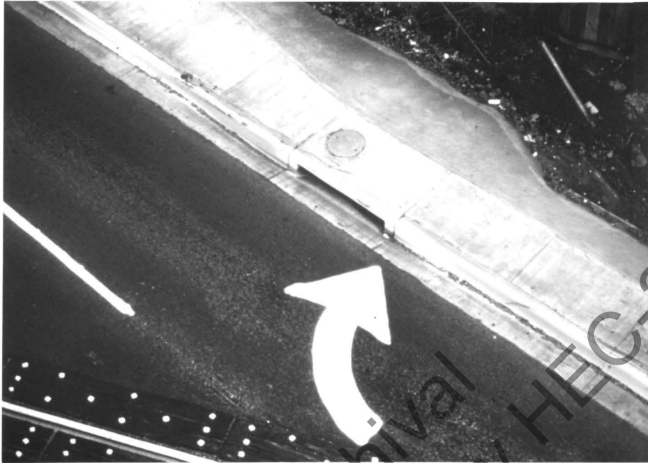
Figure 17. Depressed curb-opening inlet.
