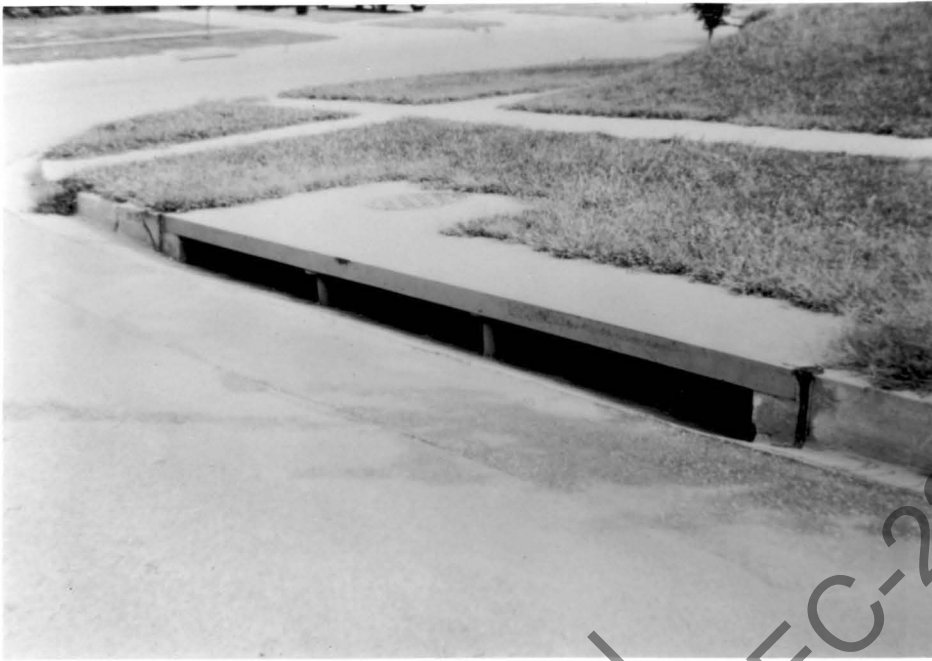
Figure 14. Curb-opening inlet with intermediate top slab supports.
