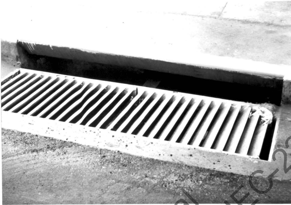
Figure 19. Combination curb-opening, 45° tilt-bar grate inlet.
