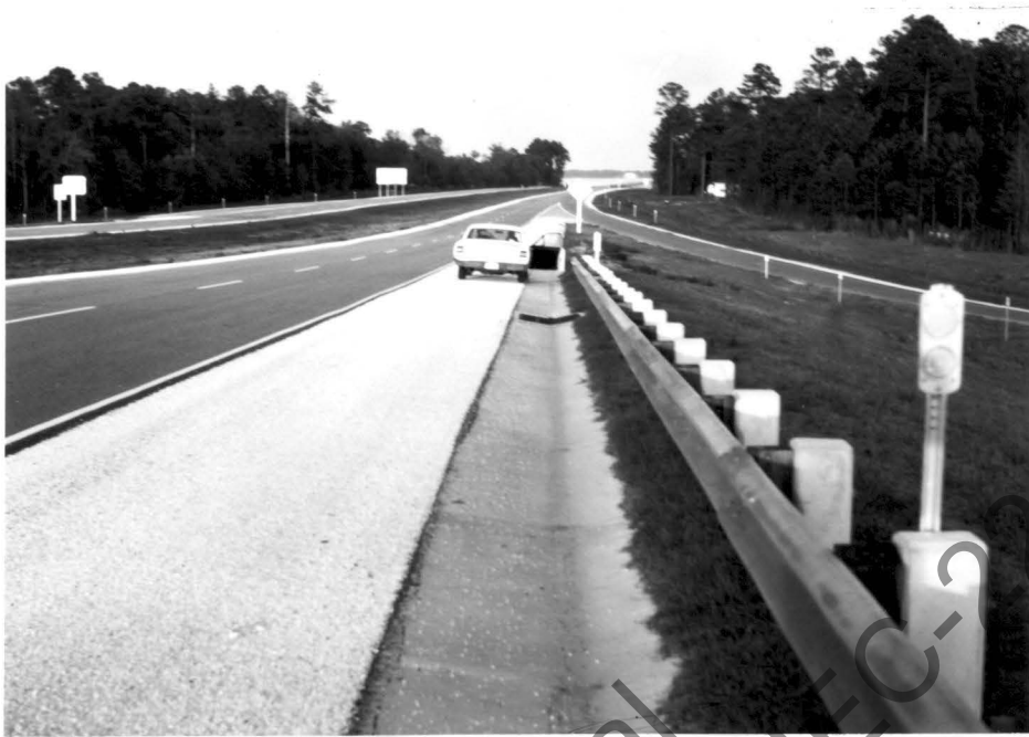
Figure 4. Use of a shallow swale in lieu of a curb.
